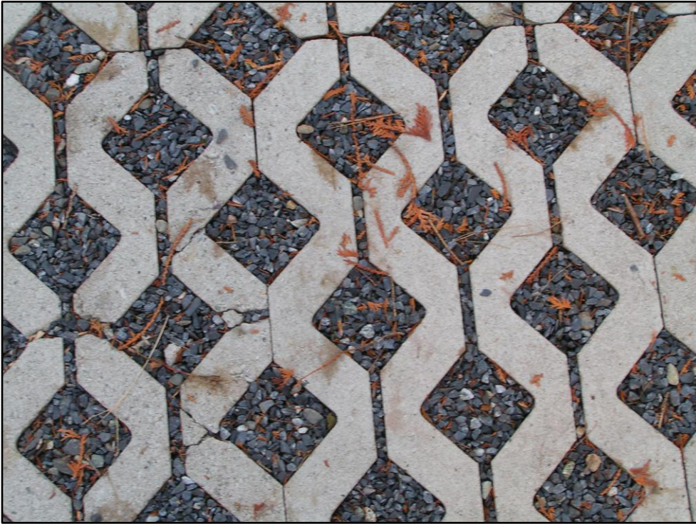
Here's a close up view of permeable pavers near Day's Store.
