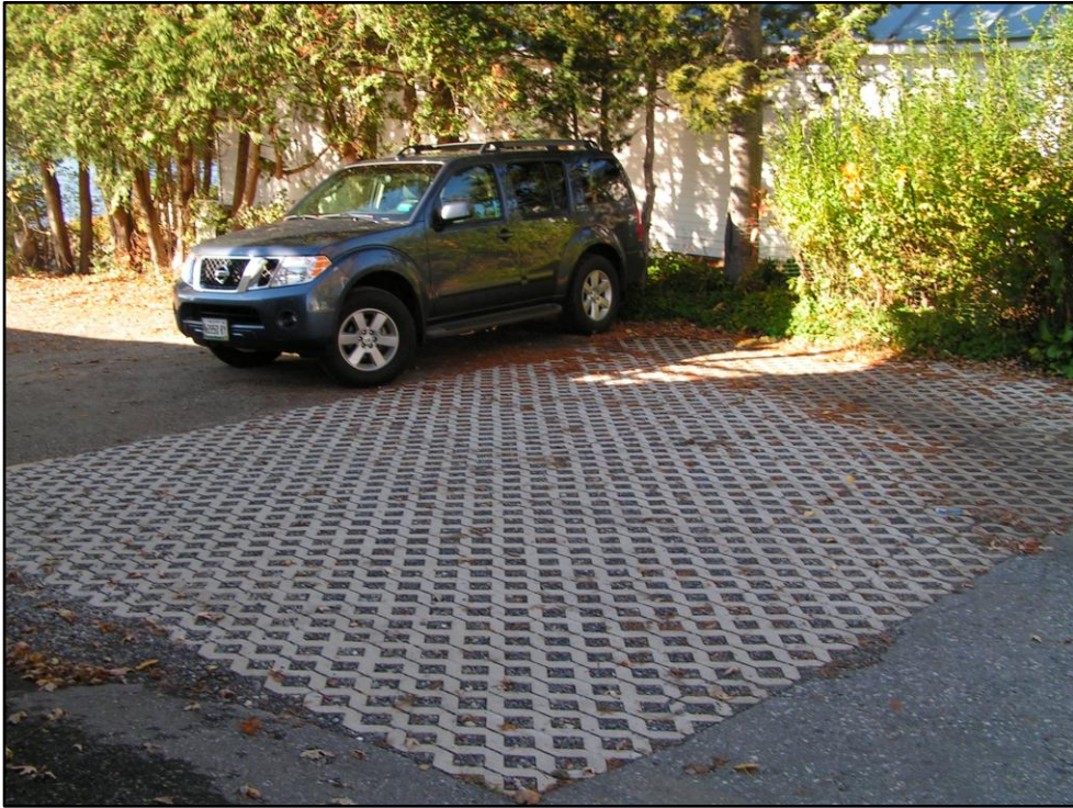
Here's another view of the porous pavers at Day's Store.
