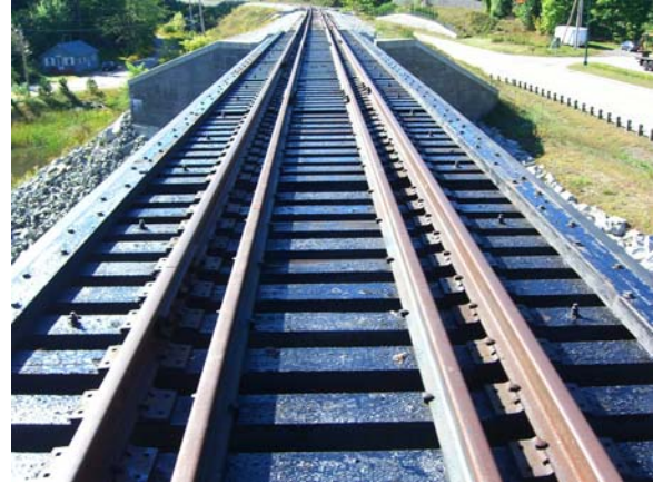
Figure 3-45 – Bridge deck, looking east
