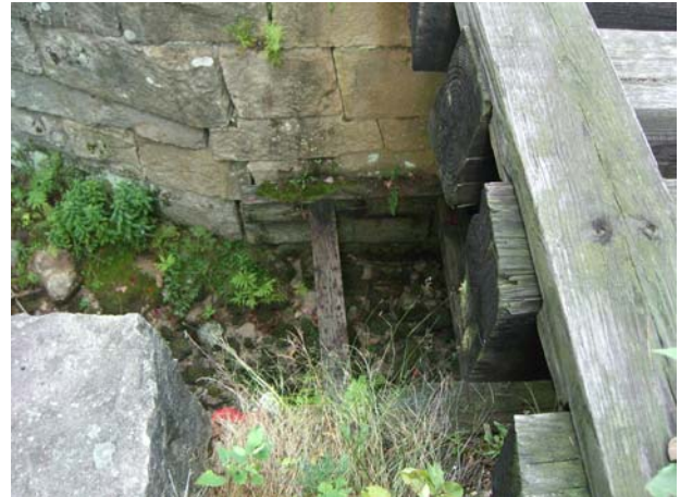
Figure 3-28 – Southwest corner of abutment
