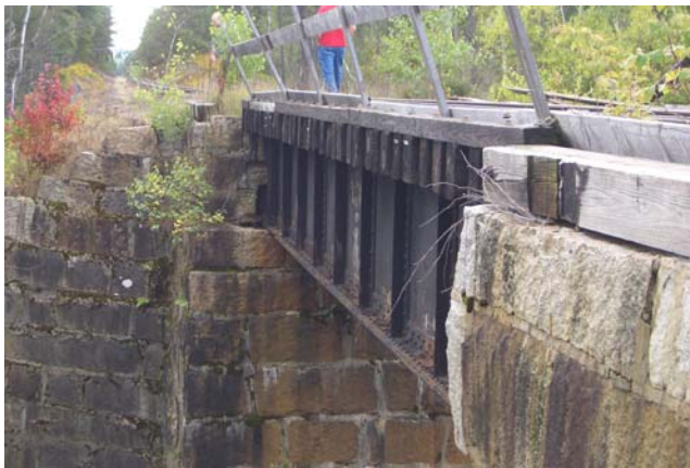
Figure 3-31 – North side of bridge, looking east
