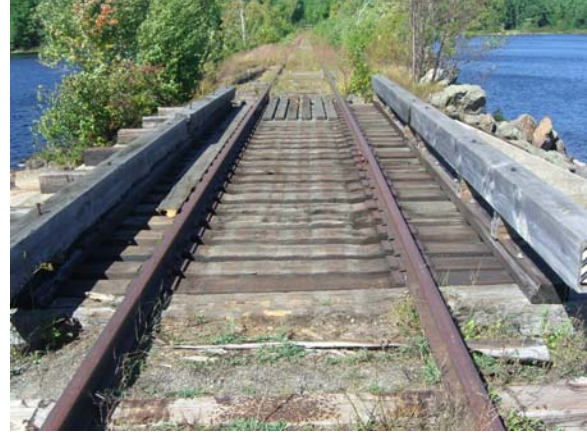
Figure 3-12 – Bridge deck, looking east
