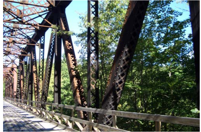
Figure 3-38 – Through trusses, looking northwest
