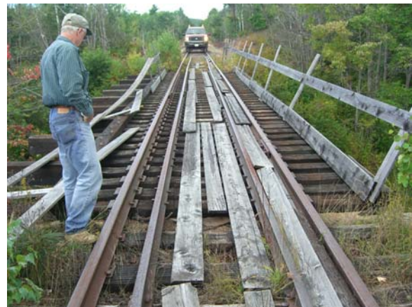
Figure 3-32 – Bridge deck, looking west
