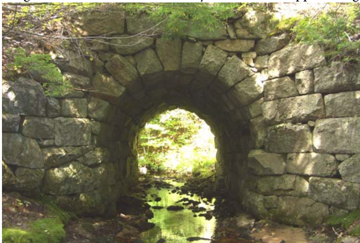
Figure 3-46 – South side of culvert
