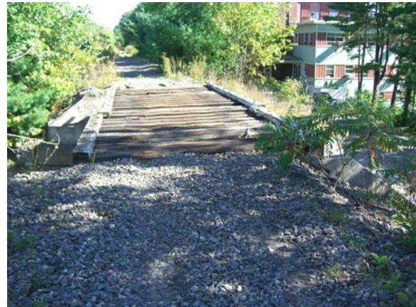
Figure 3-10 - Bridge deck, looking east. Tracks have been removed in this segment.
