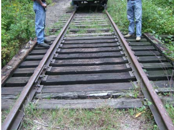
Figure 3-17 – Deck Of Bridge 30.39
