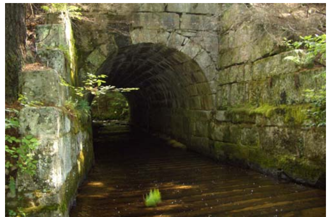
Figure 3-50 – View through length of culvert
