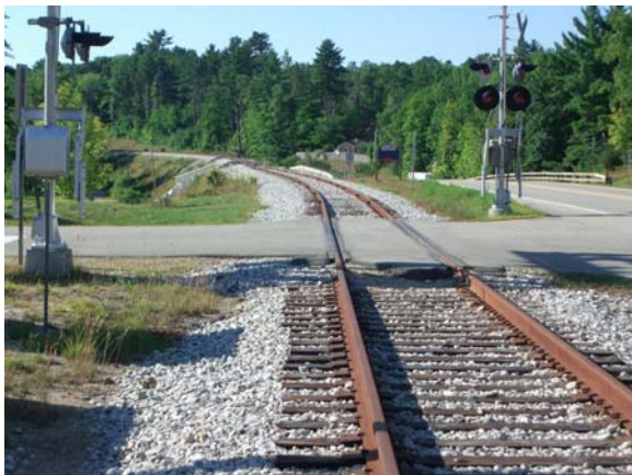
Figure 2-18 – New rubber rail seal and bituminous crossing in N. Conway, NH
