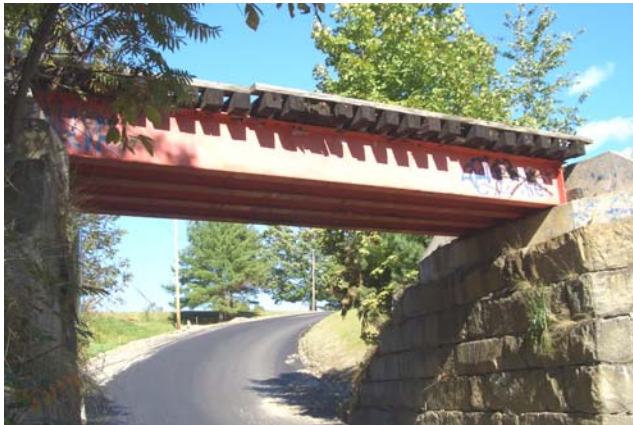
Figure 3-9 - South side of Bridge
