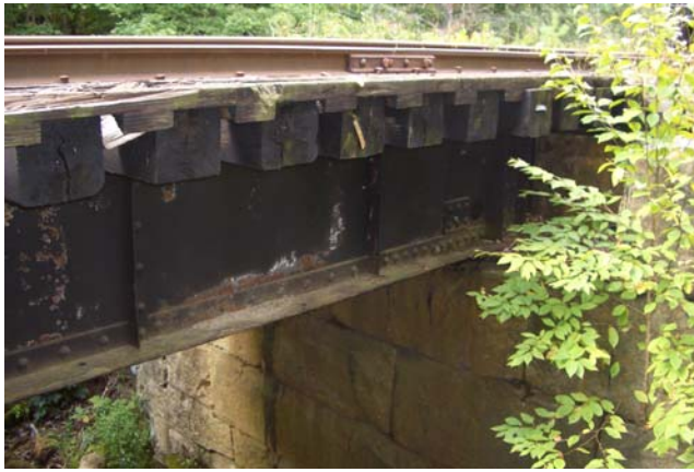
Figure 3-27 – North side of bridge
