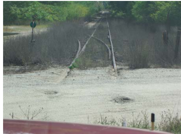
Figure 2-17 – Typical gravel crossing
