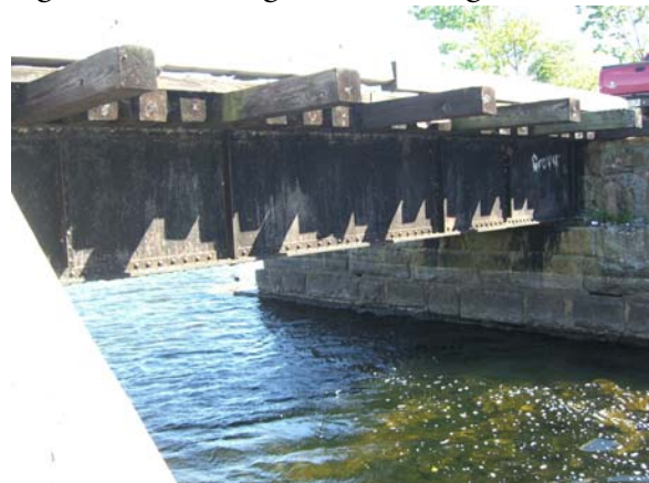
Figure 3-14 – South side, looking east
