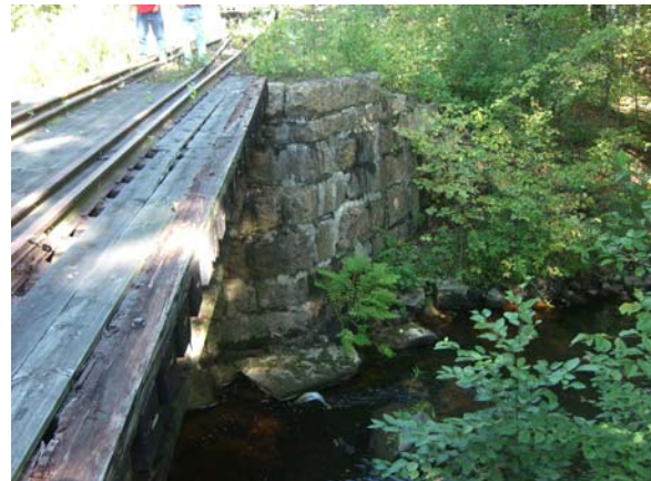
Figure 3-36 – Bridge deck and wingwall
