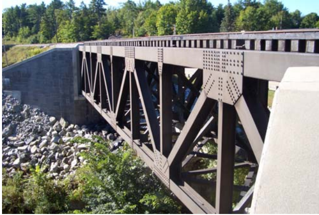
Figure 3-44 – Artist Falls Bridge – side view of truss
