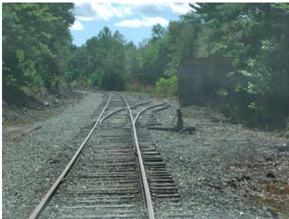
Figure 2-3 – Crushed Stone Ballasted Segment
