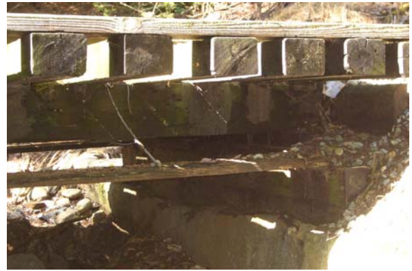
Figure 3-22 – Detail, west abutment
