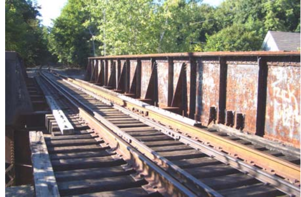
Figure 3 - Brown Street, Looking West
