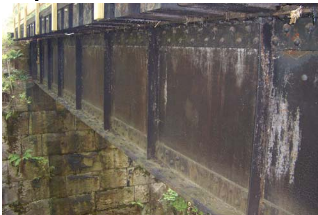
Figure 3-15 – South side, looking west
