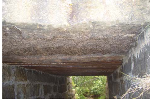
Figure 3-30 – Steel beams back inside past the granite lintel.
