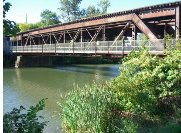
Figure 3-2 - Presumpscot River, south side. Note pedestrian bridge supported on this side.
