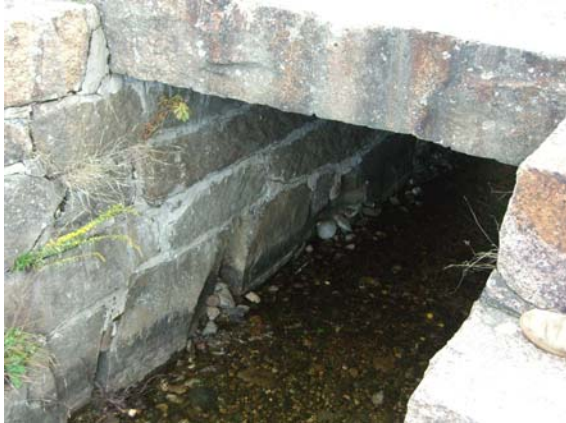
Figure 3-29 – South end of culvert
