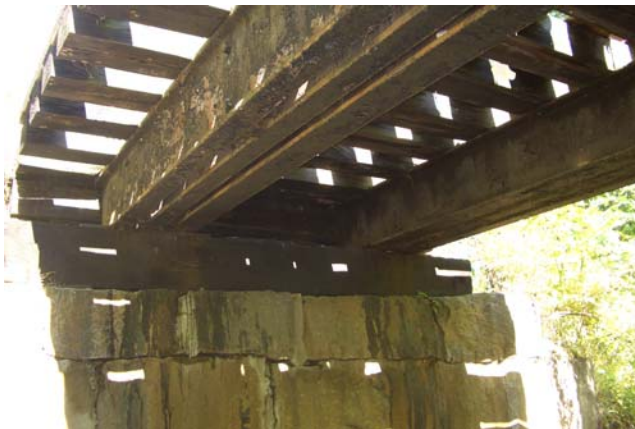
Figure 3-23 – Underside of Red Mill Brook
