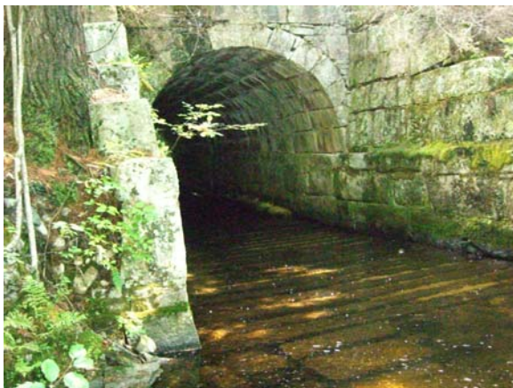
Figure 3-49 - South side of culvert Note timber grillage in stream bed
