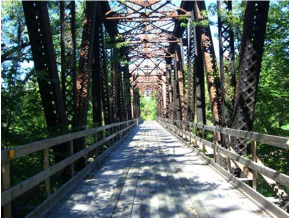
Figure 3-37 – Through trusses, looking west
