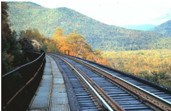
Figure 1-4 – View from Frankenstein Trestle (Named after a painter of the region and not the character in Kate Shelly's novel)
