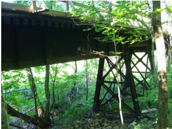
Figure 3-41 – Side view of portion of east approach trestle
