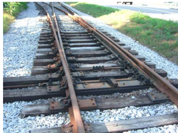
Figure 2-13 – Relay 115 RE, No. 10 Turnout installed by NHDOT in North Conway
