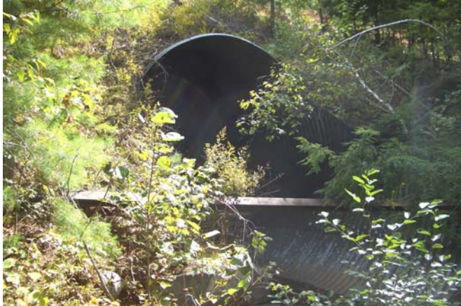
Figure 3-47 – South side of pipe culvert
