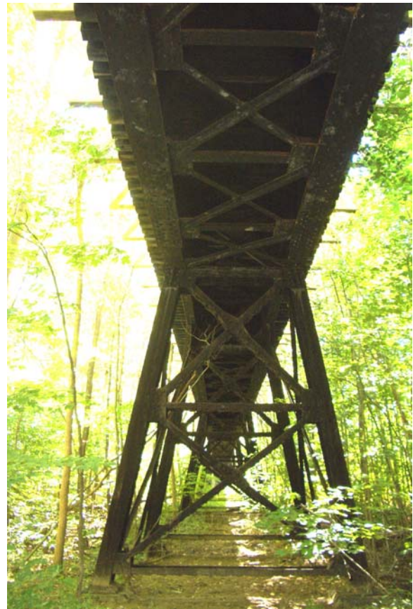
Figure 3-42 – Portion of east approach trestle, looking west
