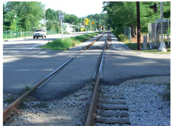
Figure 2-19 – New rubber rail seal crossing and track in N. Conway, NH
