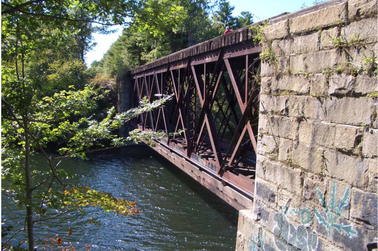
Figure 3-11 – Presumpscot River, looking west
