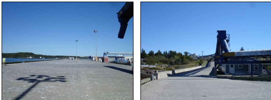
Figure 4: Pier Deck and Access Ramp 7
