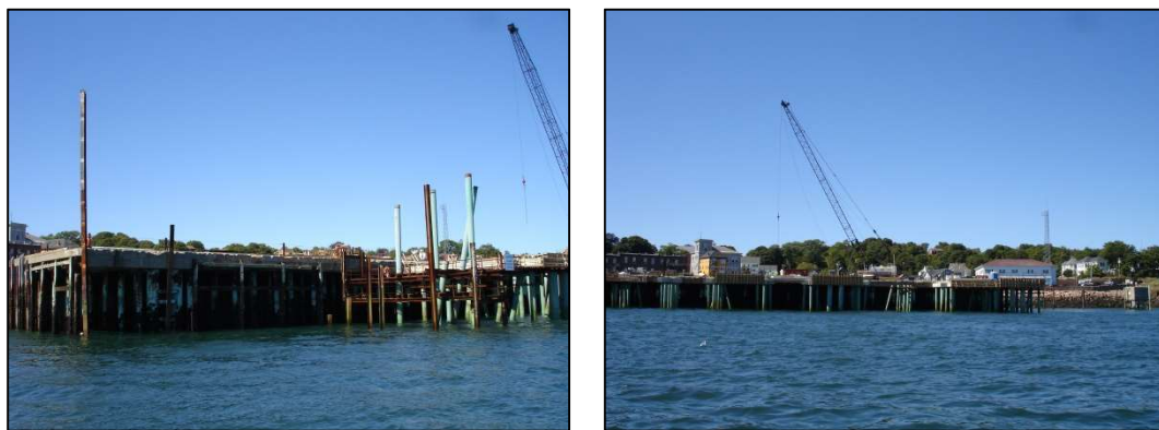
Figure 10: Breakwater Terminal Reconstruction 14
