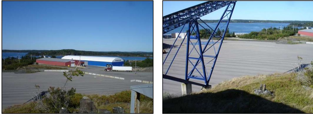
Figure 5: Storage Sheds and Open Storage Area 8
