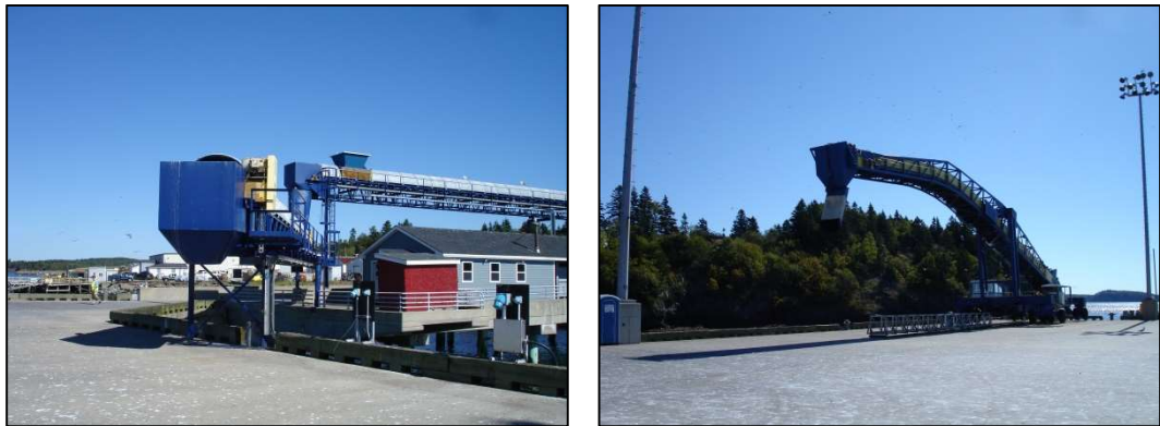
Figure 6: Conveyor System and Ship Loader 10
