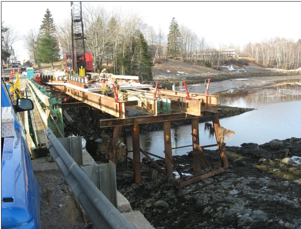
Figure 3-35. Typical trestle/temporary bridge construction.
