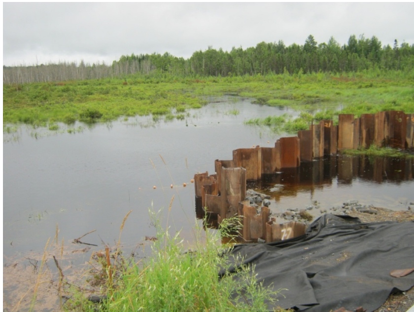
Figure 3-8. Sheet pile used as a cofferdam (upstream of work area).
