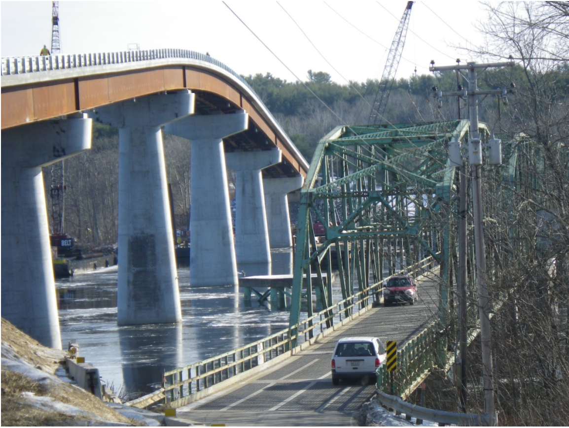
Figure 3-25. The Richmond-Dresden Bridge over the Kennebec River is constructed with cast-in-place, concrete, spread footing piers.
