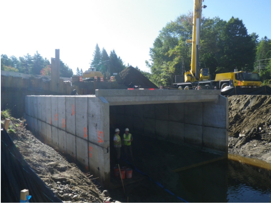
Figure 3-18. Setting a 26-foot wide concrete box structure.
