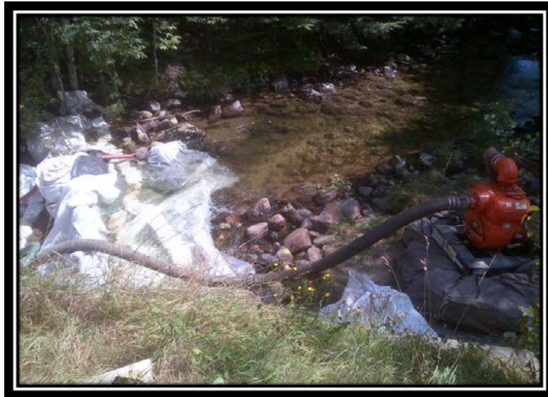
Figure 3-12. A pump sending upstream water around a cofferdam.
