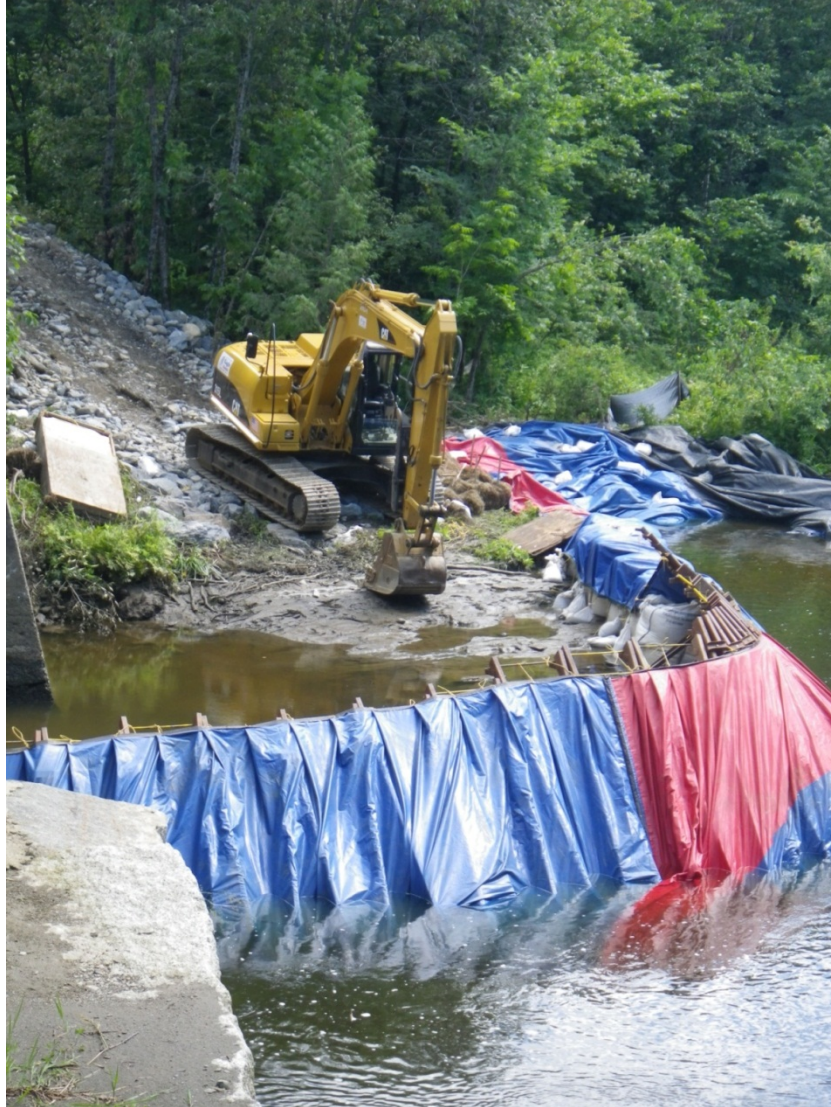
Figure 3-9. Work behind a Portadam® cofferdam.
