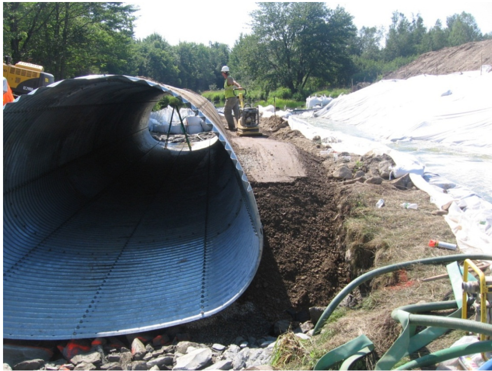
Figure 3-19. Bedding a corrugated metal culvert.
