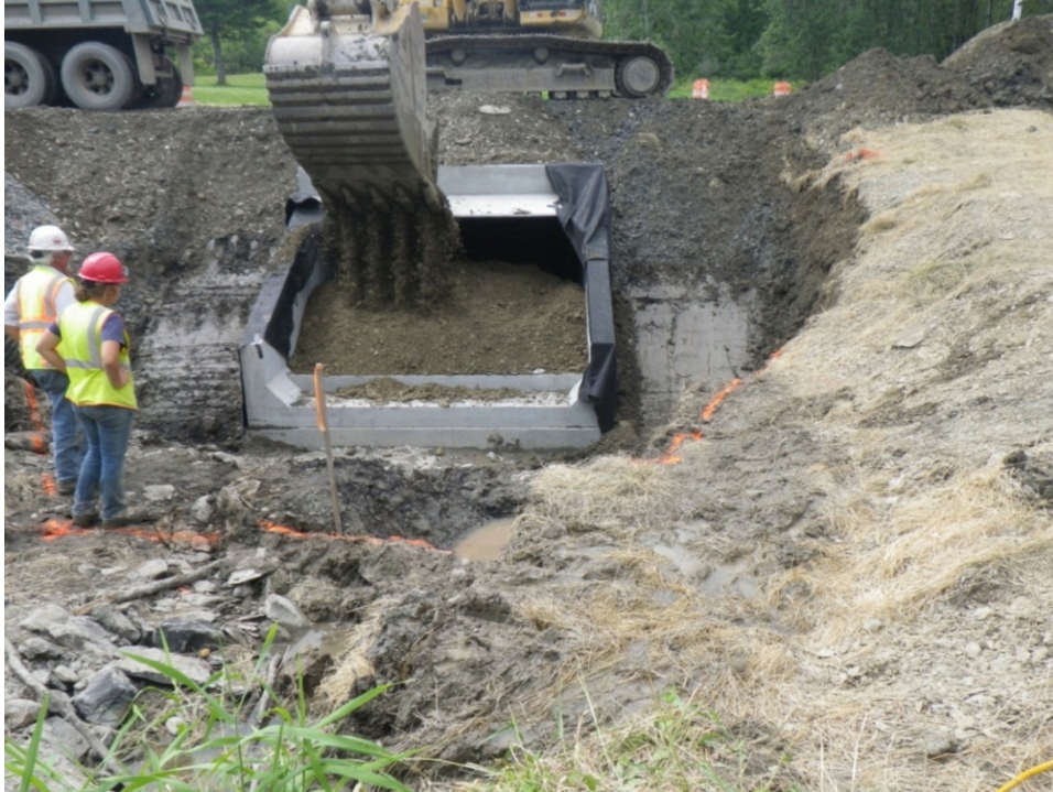
Figure 3-20. Concrete box structure being backfill and receiving bedload.
