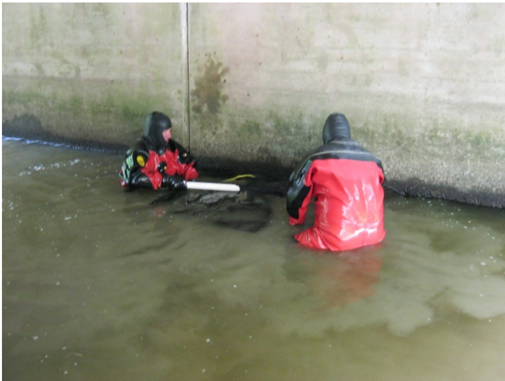
Figure 3-33. Grout bag repair at a bridge in Maine.
