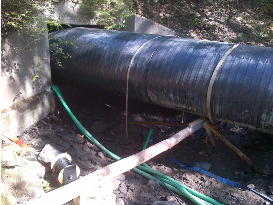
Figure 3-38. Slip line being inserted.
