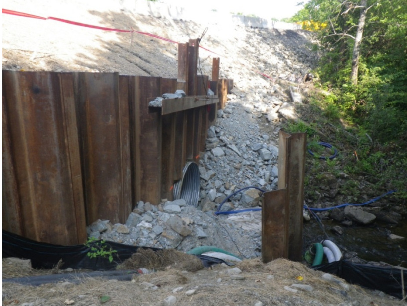
Figure 3-7. Sheet pile used as a cofferdam (upstream of work area).
