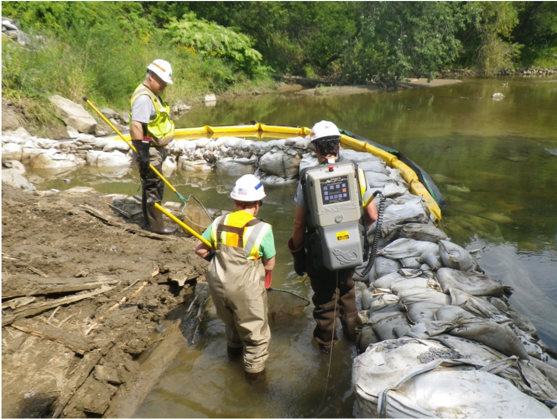
Figure 3-5. Example of a cofferdam constructed of small sandbags.
