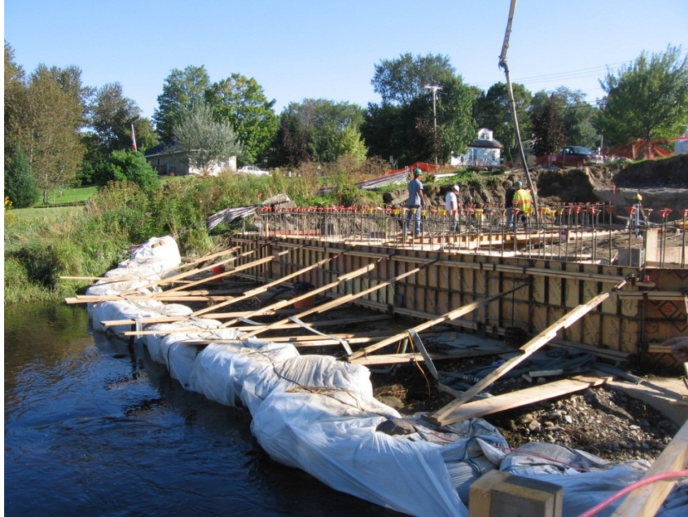
Figure 3-21. Bridge abutment construction behind a cofferdam constructed of industrial sandbags
