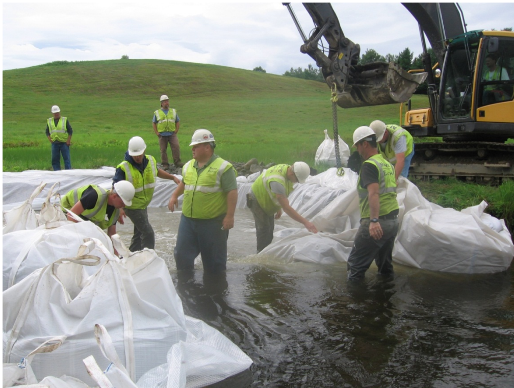
Figure 3-3. Placement of plastic sheeting under sandbag cofferdam.
