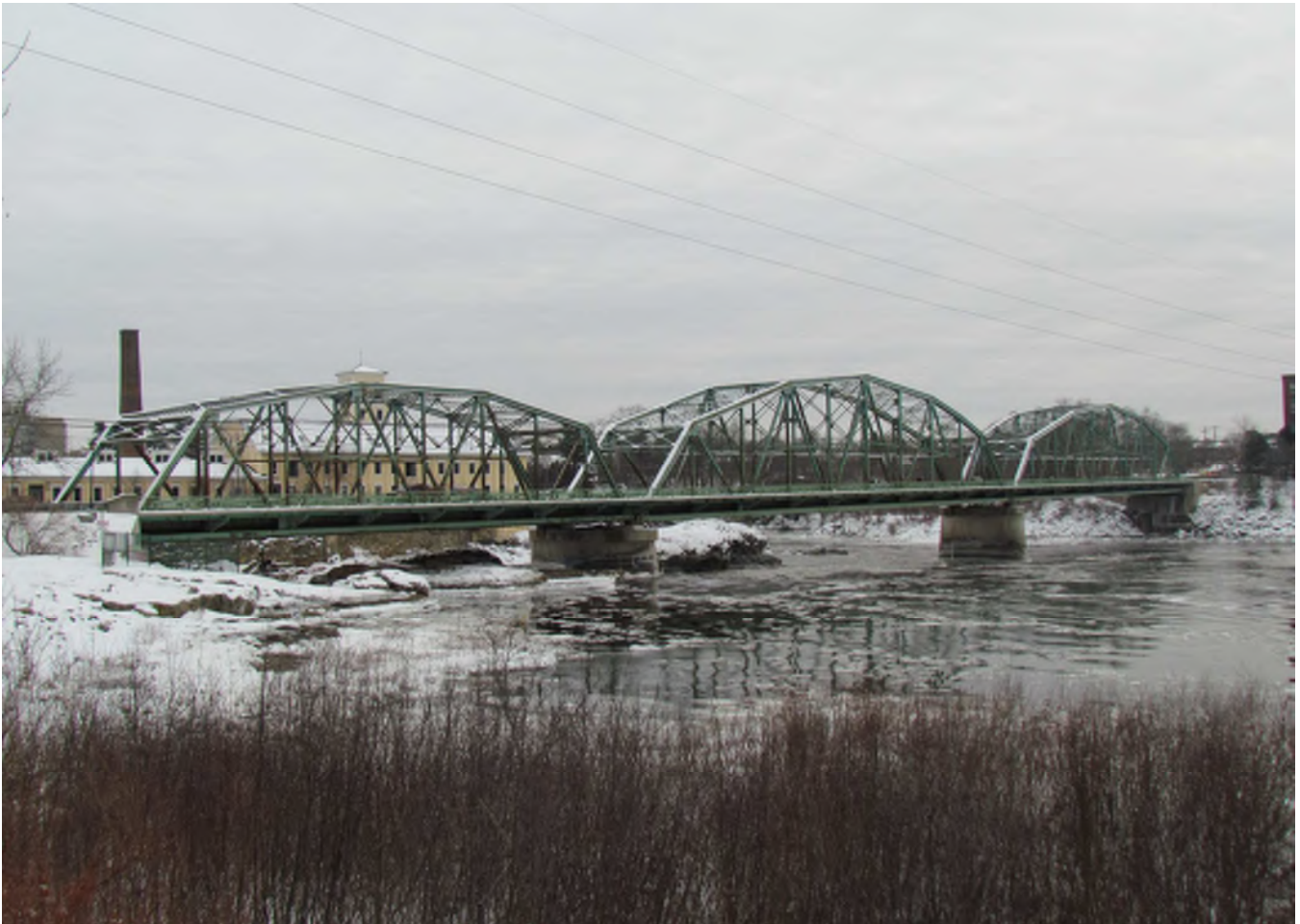
Frank J Wood Bridge, February 2016
