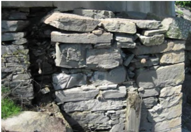
Figure 12: Abutment masonry
