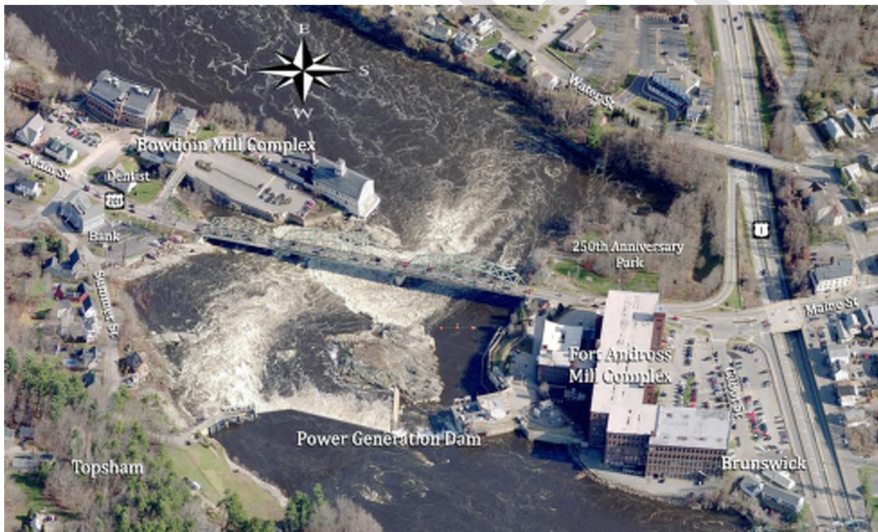
Figure 1: The Frank J. Wood Bridge spanning the Androscoggin River between Brunswick and Topsham
