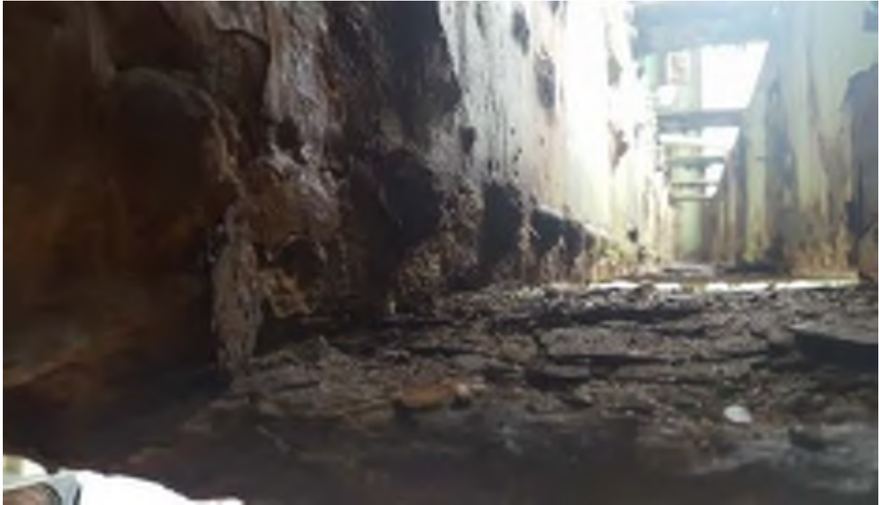
Figure 11: Bottom chord corrosion and debris
