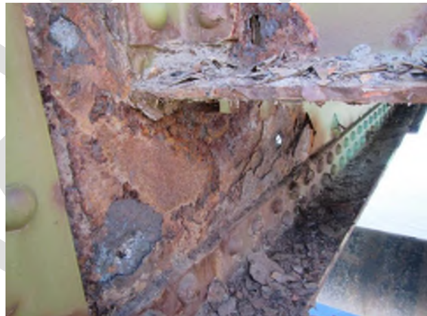
Figure 9: Deteriorated floorbeam
