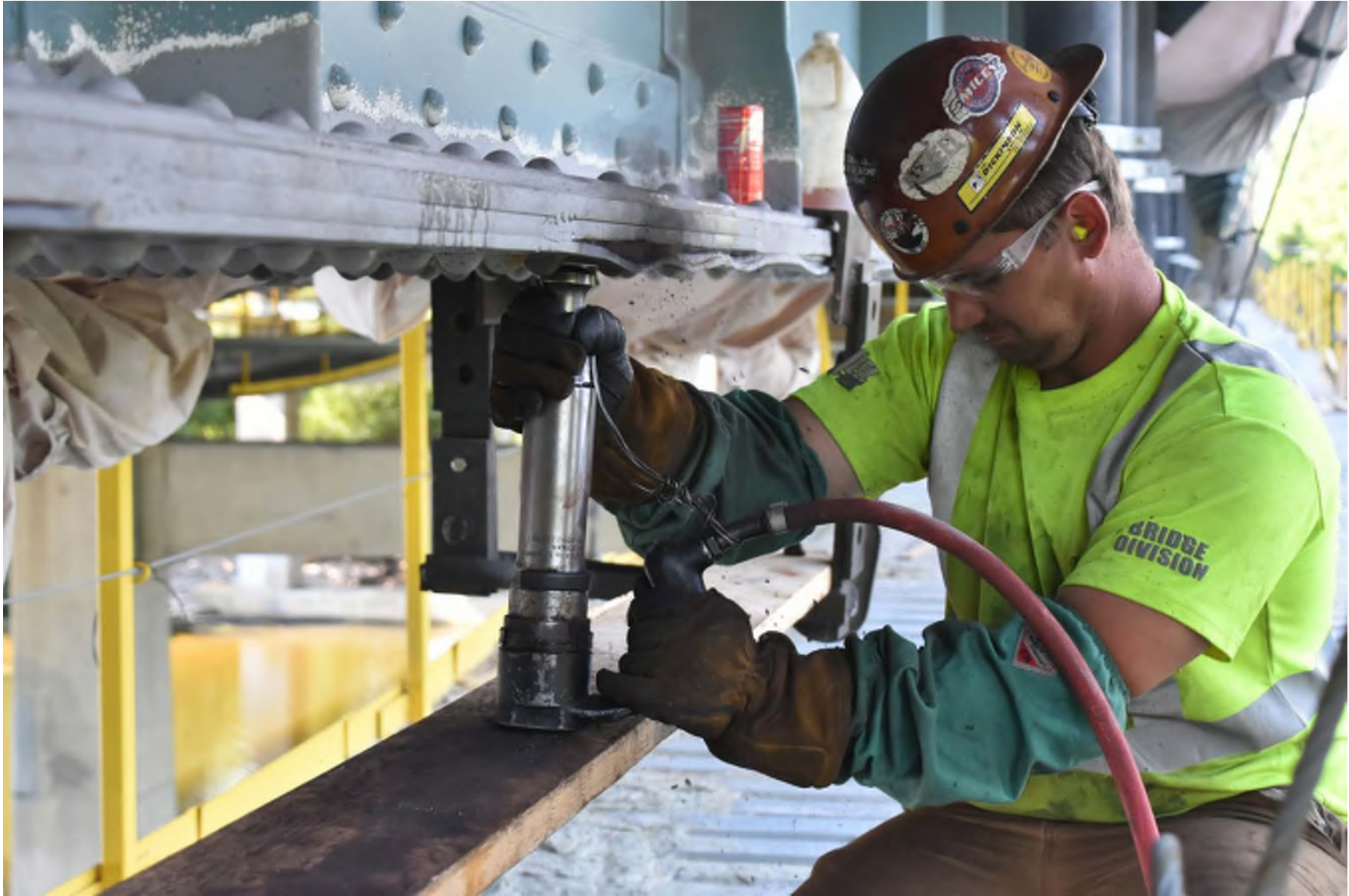
Driving the pack rust out.
