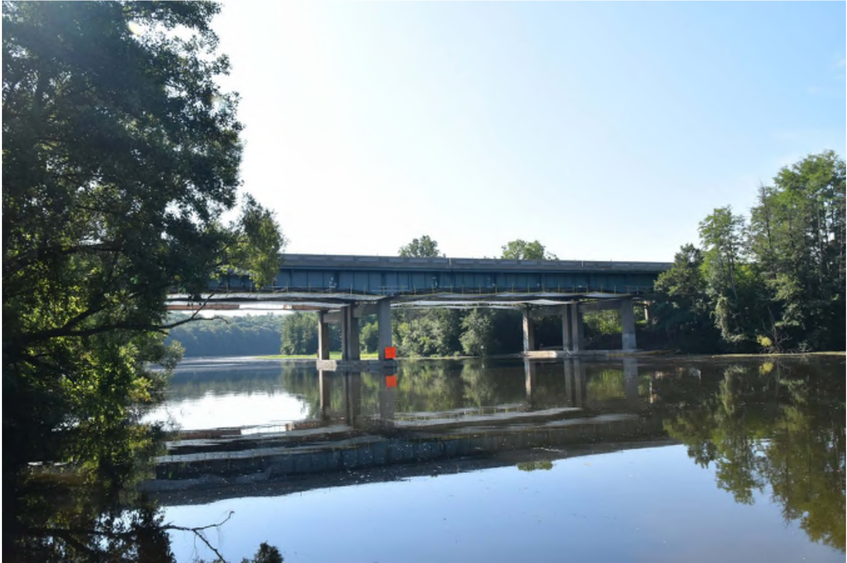
Overview of bridge.
