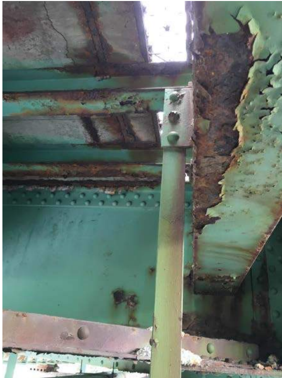
Photo #25: Typical view of bottom flange of S3 & S8 in spans 1 & 2 (8/1/16)
