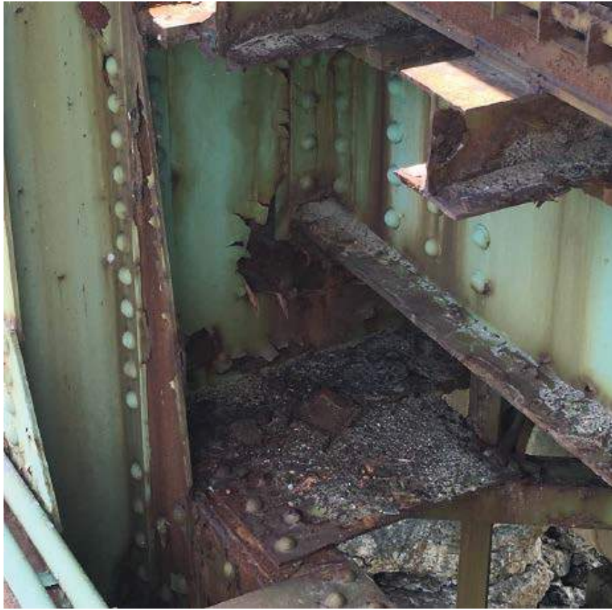
Photo # 21: General view of floor beam end in span 3 (8/2/16)
