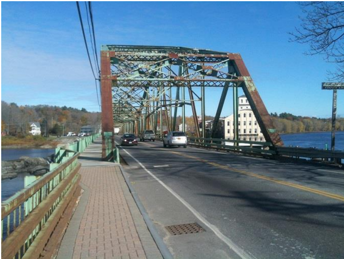
Photo #1: Bridge View looking north from Brunswick
