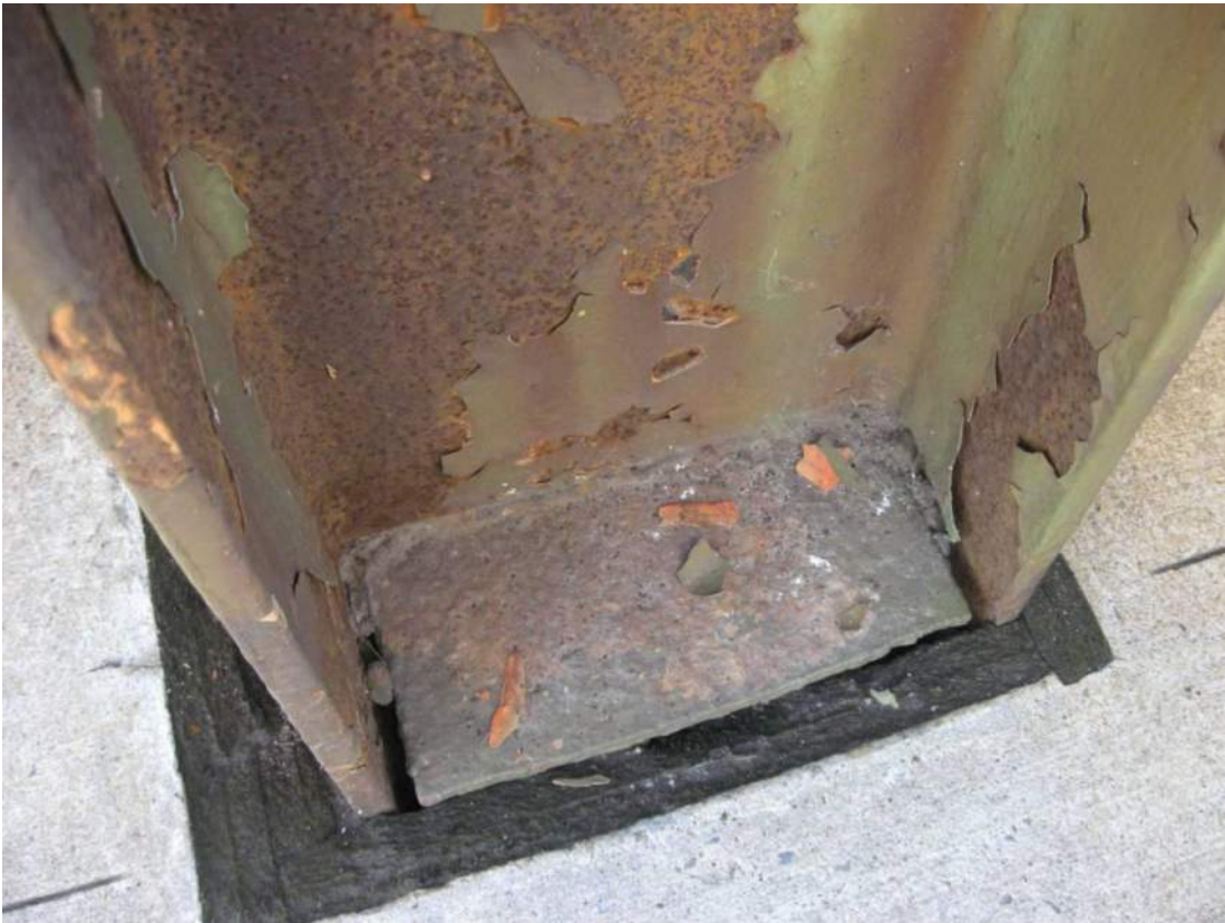
Photo 37 – Sidewalk truss verticals and diagonals have welded plates at sidewalk level openings. These plates represent FSD's in FCM's (wherever base members are FCM's).
