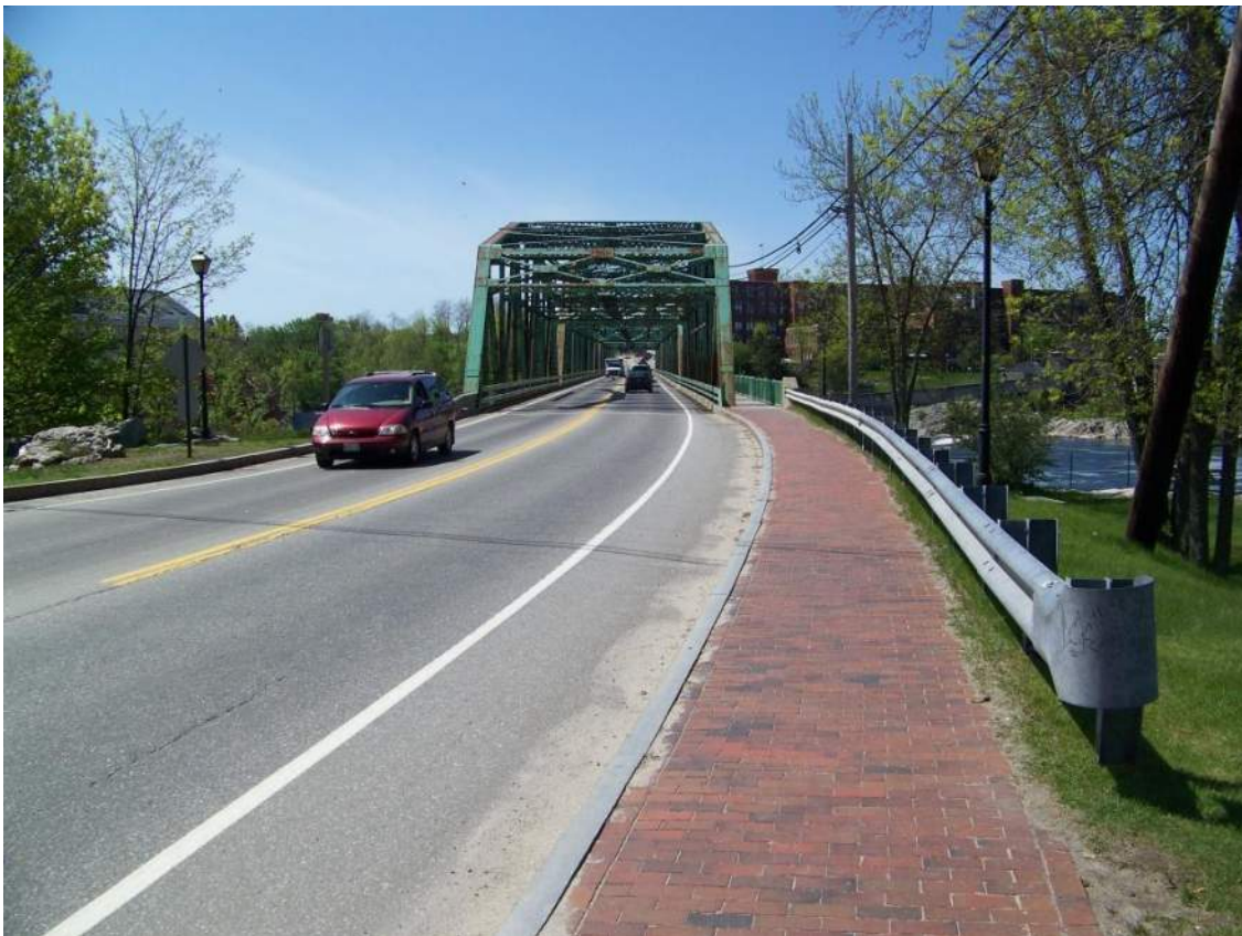
Photo 3 – View of bridge looking south from the north approach roadway.
