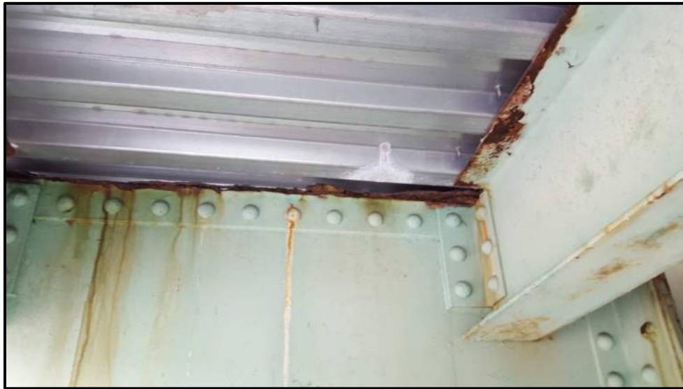
Photo A25 – View of the top half of cantilevered brackets that support the sidewalk.
