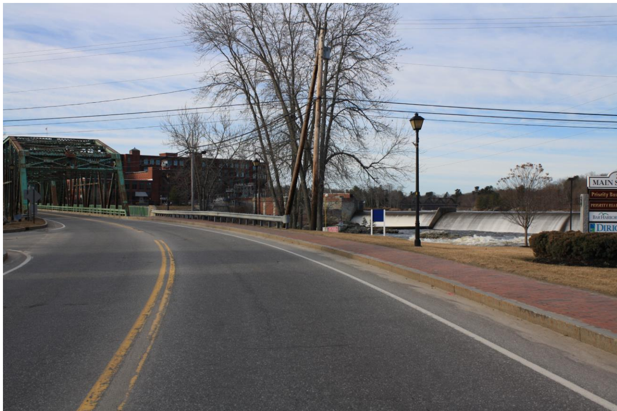
Photo #6: Topsham Approach looking south
