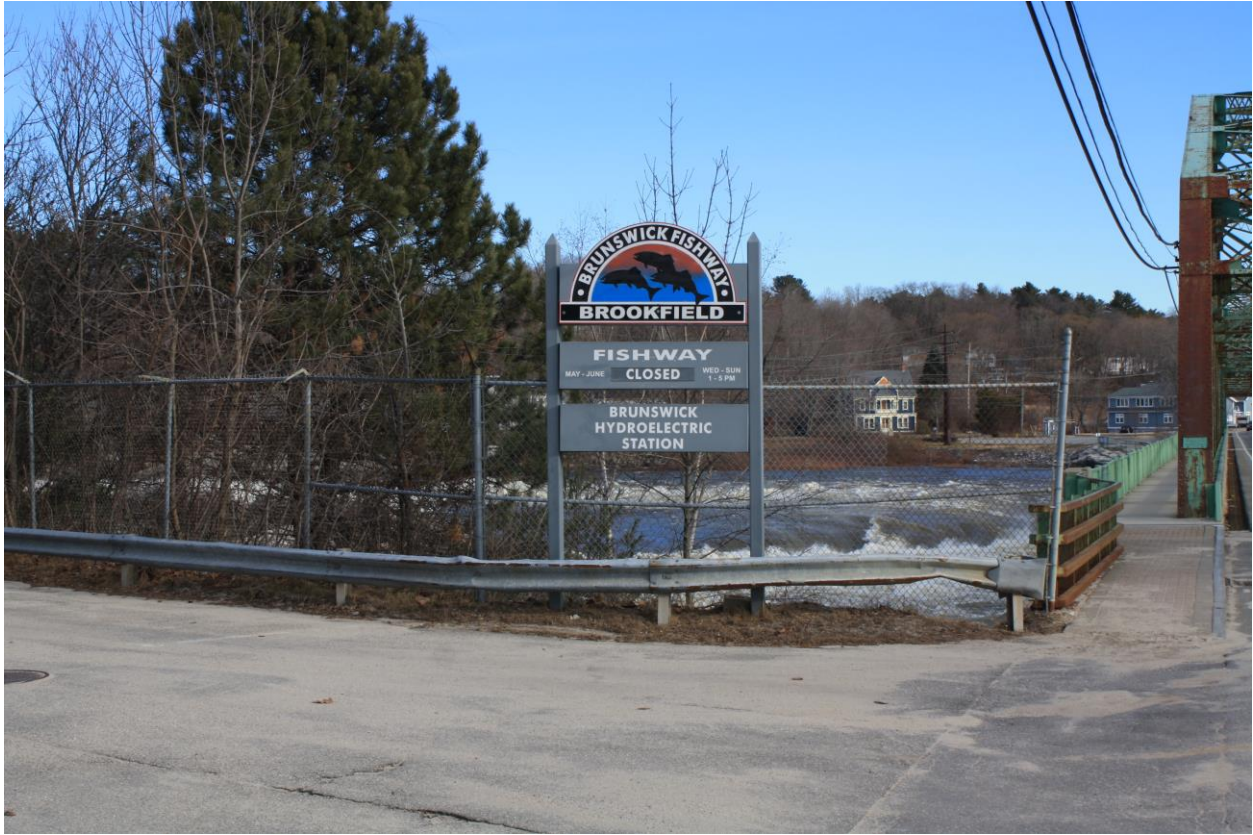
Photo #7: Brunswick Approach looking north
