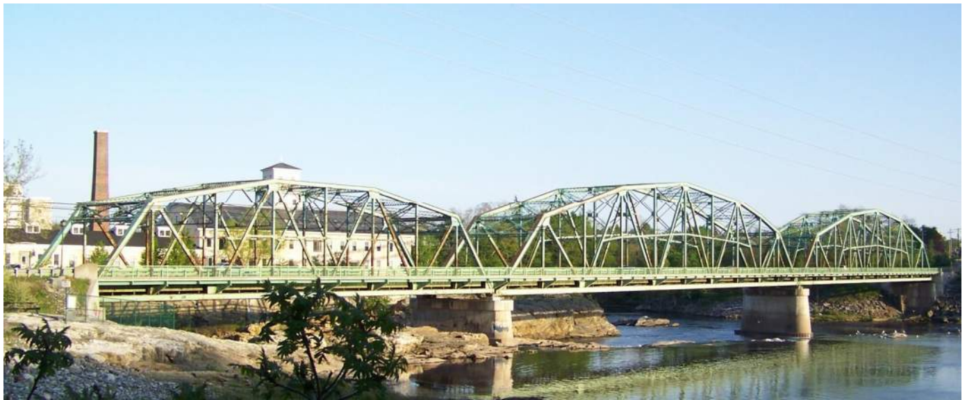
Photo 1 – Partial upstream elevation looking southeast with Span 1 at right. (Note- See Report cover for similar photo).
