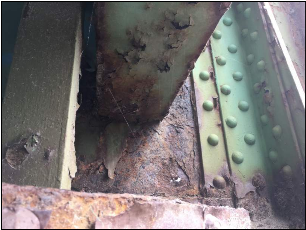
Photo A2 – Floorbeam 5, Roadway Truss @ Stringer 8 (Exterior)
