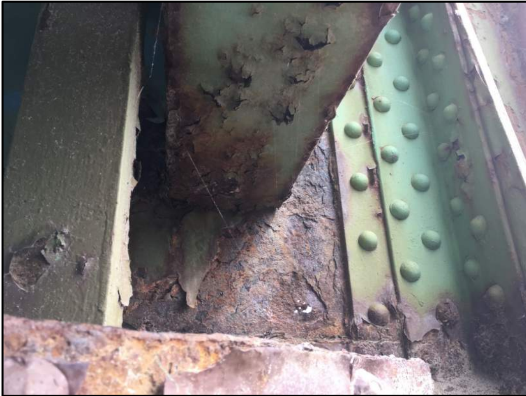
Photo A2 – Floorbeam 5, Roadway Truss @ Stringer 8 (Exterior)
