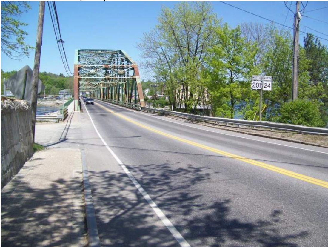
Photo 2 – View of bridge looking north from the south approach roadway. Note minor impact damage to southeast corner guiderail at right.
