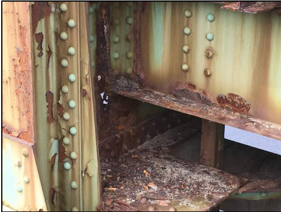
Photo A1 – Floorbeam 7, Roadway Truss @ Stringer 8 (Exterior)
