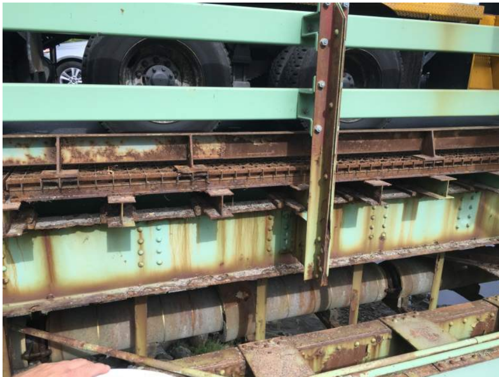
Photo #4: General view of the superstructure section (8/1/16)
