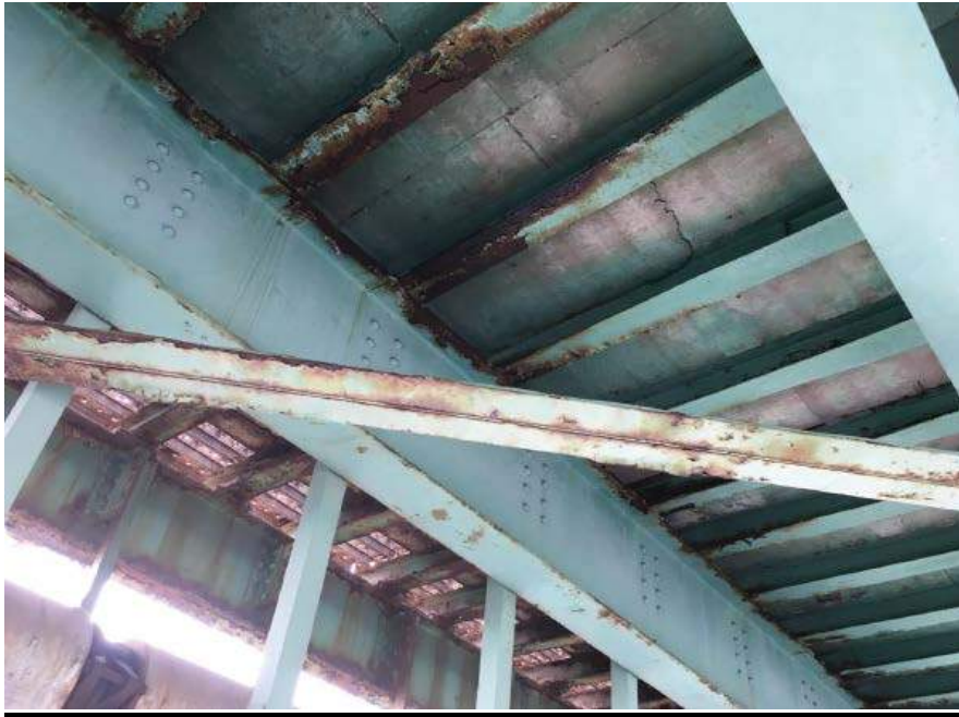
Photo #43: Typical view of cross beams (needle beams) in the first interior bays from S4 through S7 (8/1/16)
