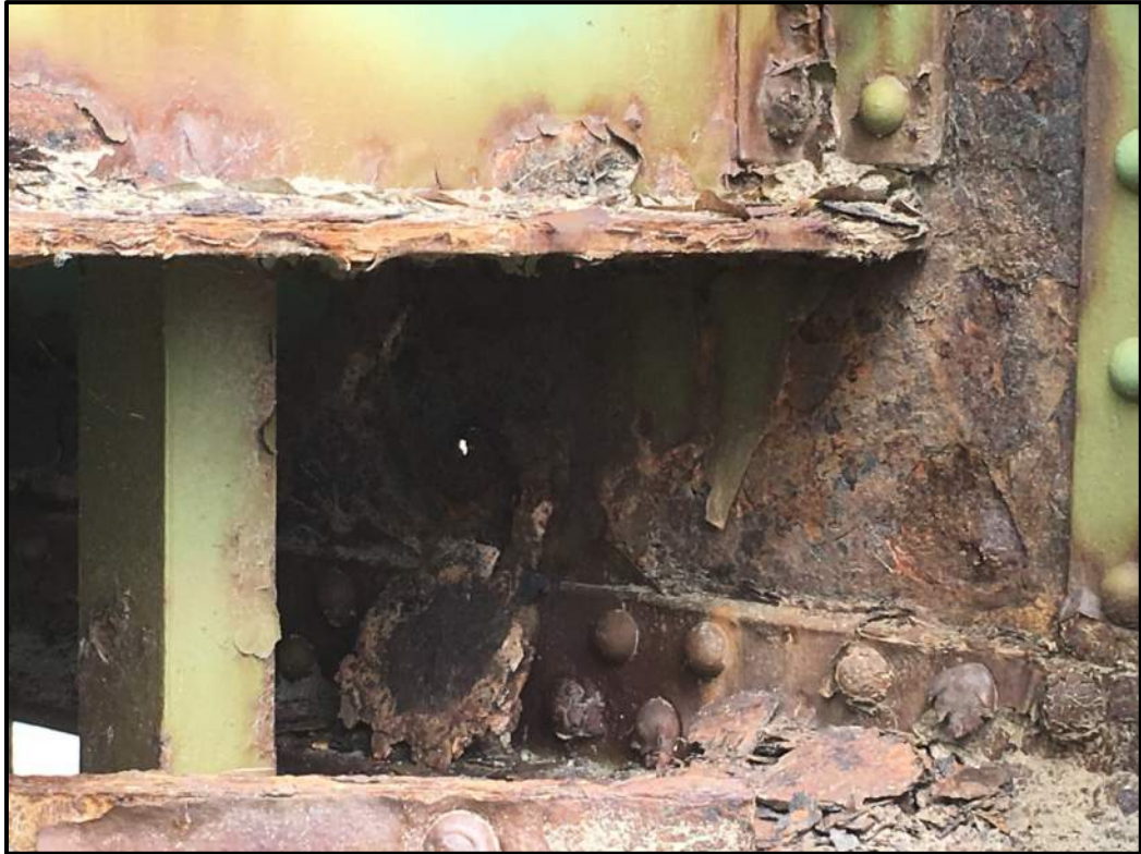
Photo A3 – Floorbeam 2, Roadway Truss @ Stringer 8 (Exterior)
