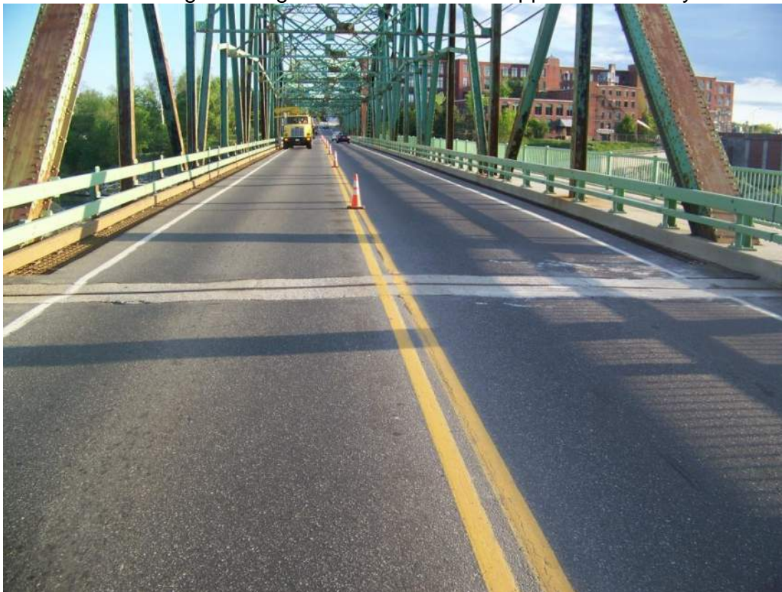
Photo 4 – General top of deck view in Spans 2 & 3, looking south from Span 3 at approximately 25 feet north of Pier 2.
