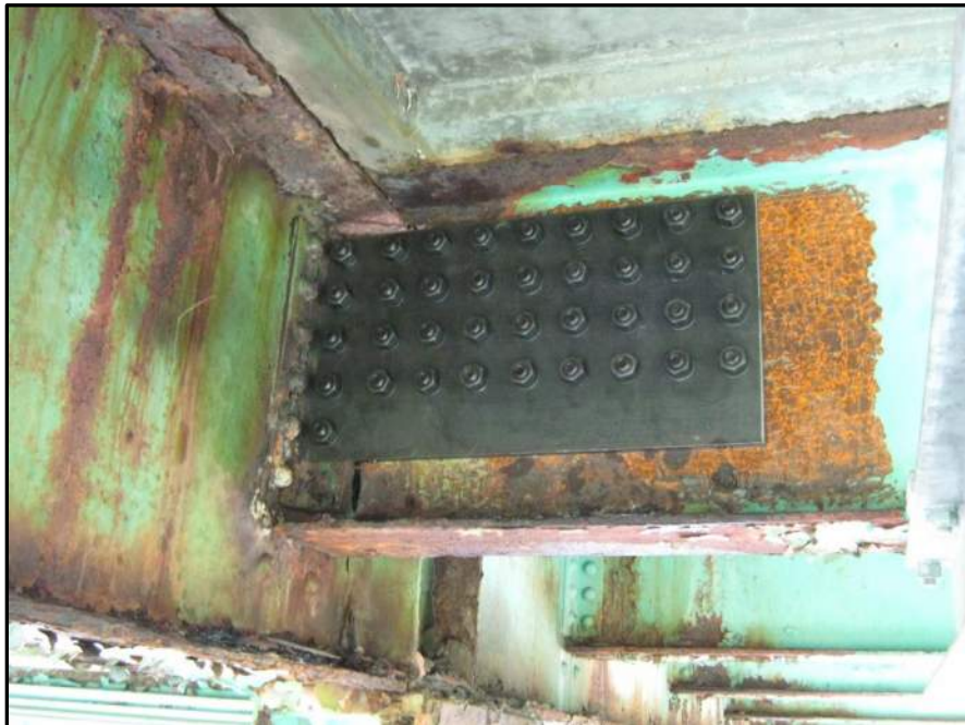
Photo A28 – End result of a typical Stringer to Floorbeam connection.
