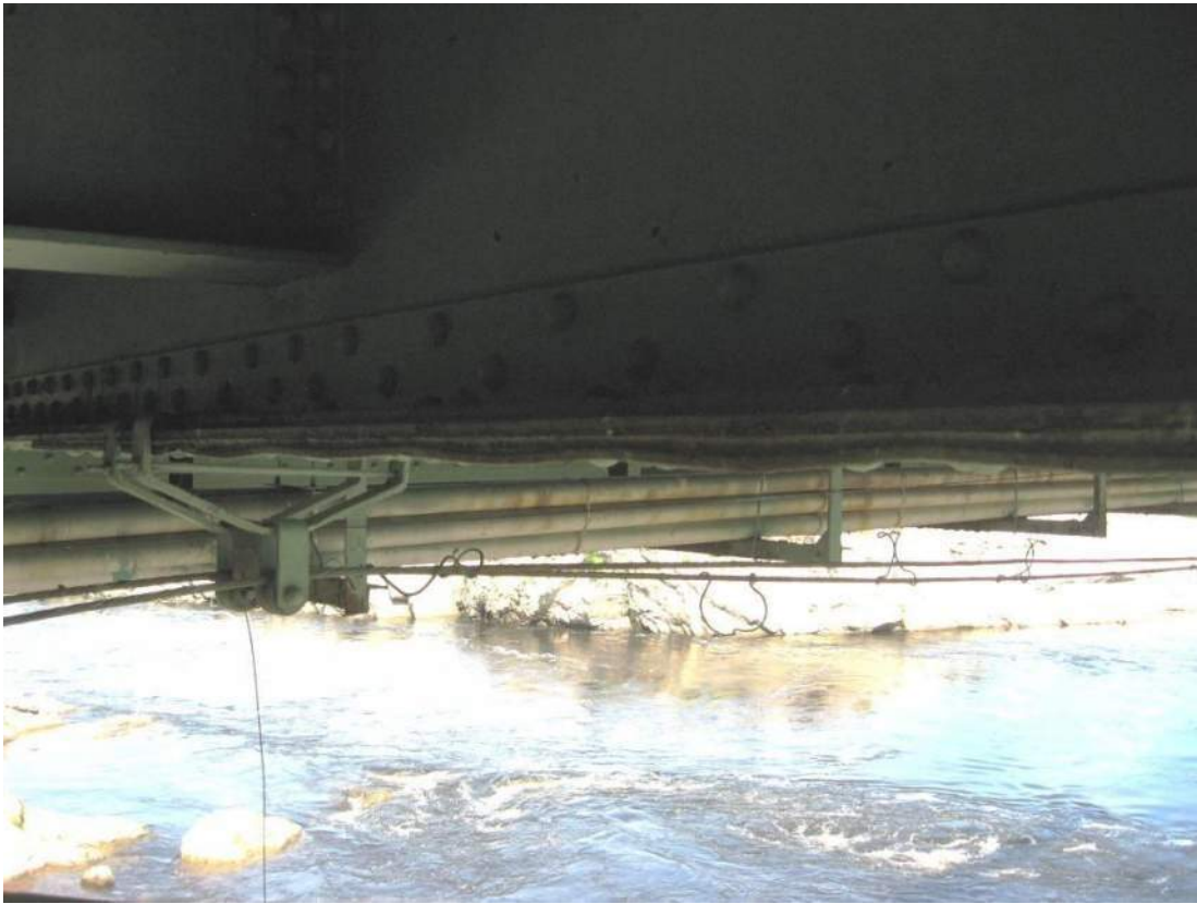
Photo 39 – Previously arrested pack rust was observed in the Span 1 FB1 floorbeam between the bottom flange cover plate and the edges of the bottom flange angles.
