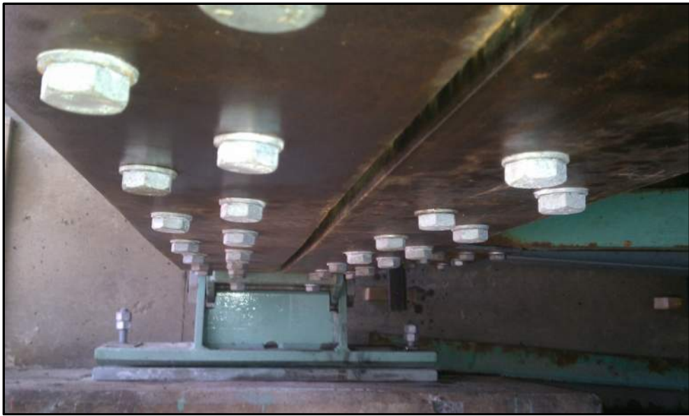
Photo A27 – End result of repair to built-up Floorbeam bottom flange.
