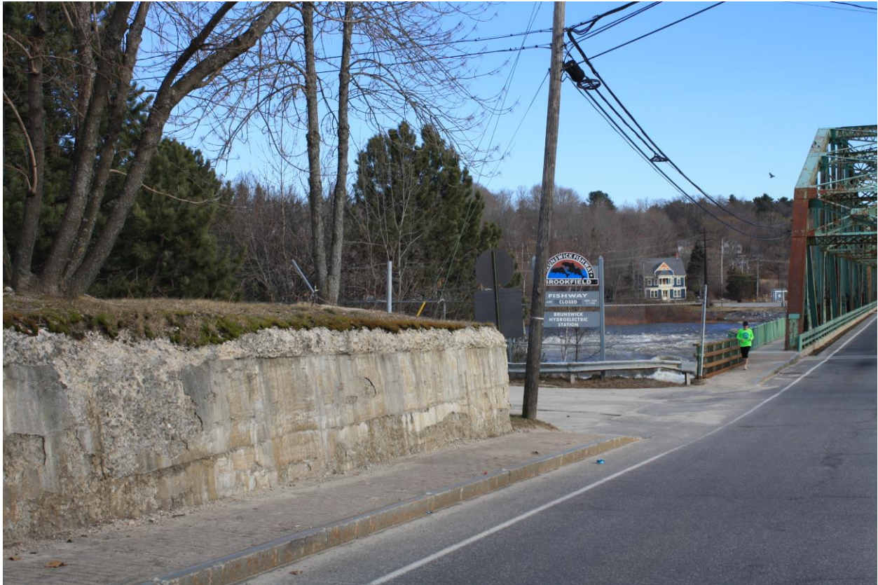
Photo #8: Fort Andross Parking Lot Wall
