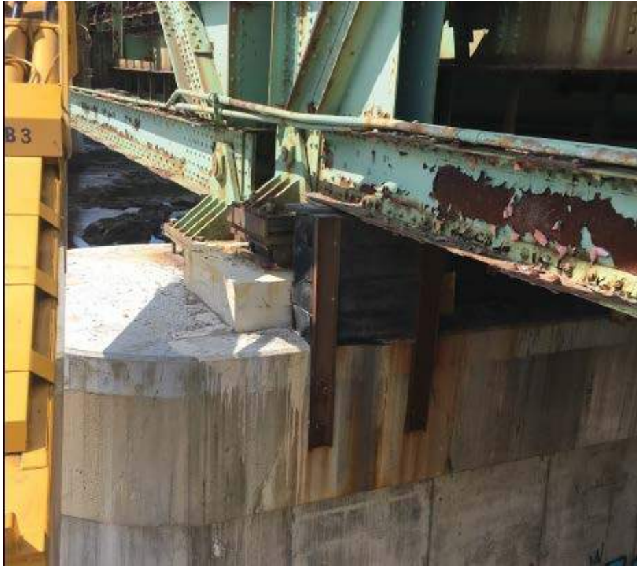
Photo #57: Shoring of non-sidewalk bearing, pier 2, span 3 (looking southwest) (8/2/16)
