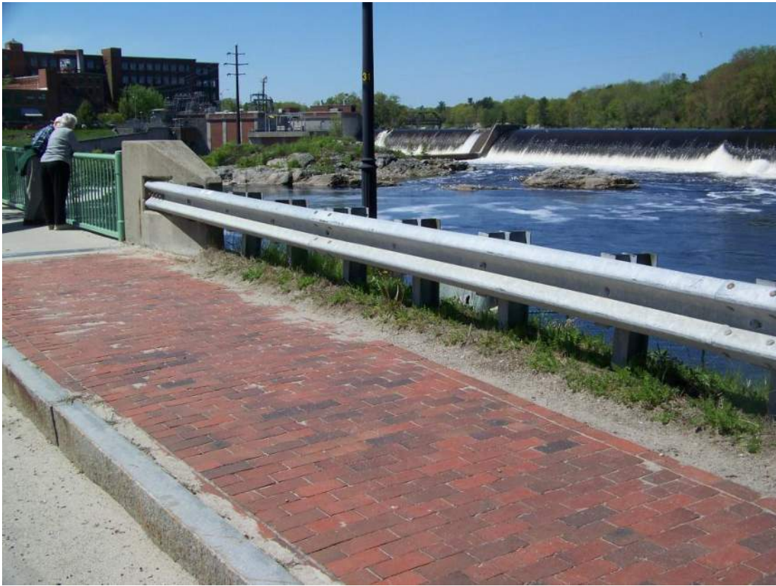
Photo 87 – The approach guidrail at the northwest corner of the bridge is aligned with the outboard edge of the sidewalk and connected to the west pylon.
