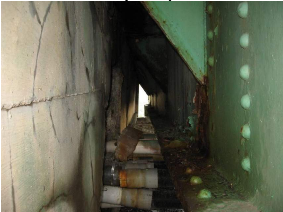
Photo 80 – There is a large 3 foot by 3 foot by 3 inch deep spall in lower portion of backwall around edges of utility conduit penetration and extending behind sidewalk truss.
