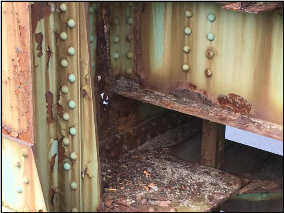
Photo A1 – Floorbeam 7, Roadway Truss @ Stringer 8 (Exterior)
