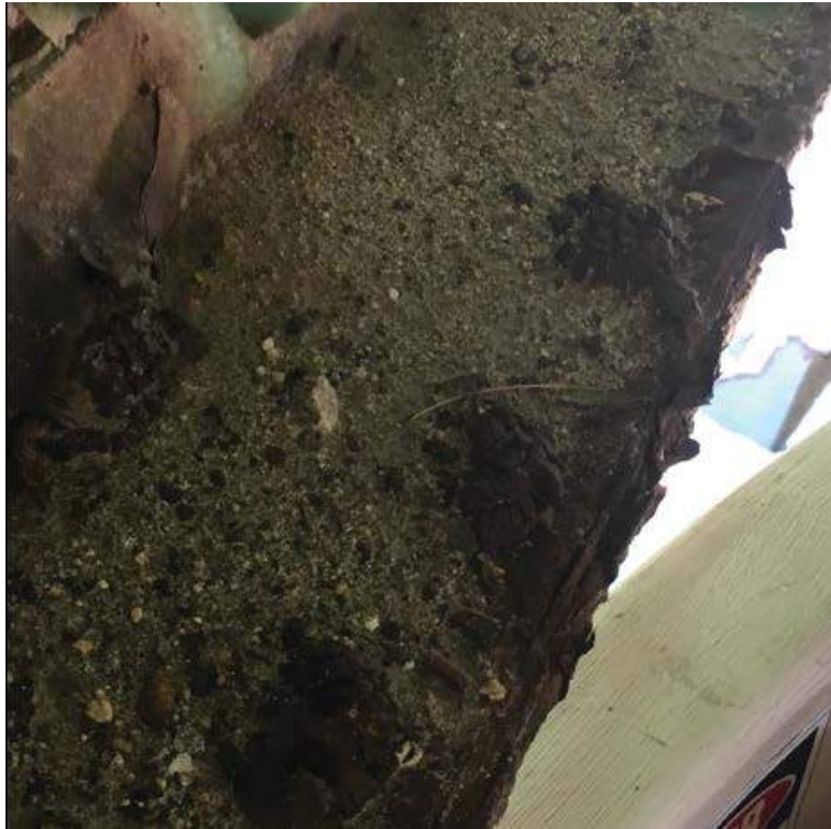
Photo #39: Remnants of rivet heads along the top of the bottom flange of the bottom chord of the sidewalk truss (western) in span 3 (8/2/16)
