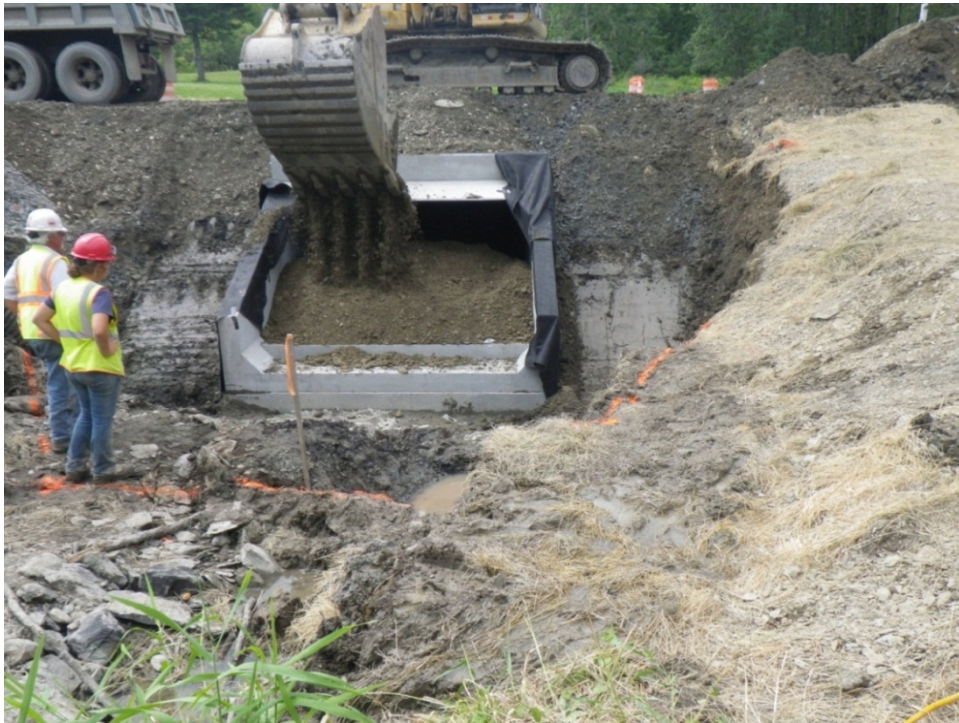
Concrete box structure being backfilled and receiving bedload.
