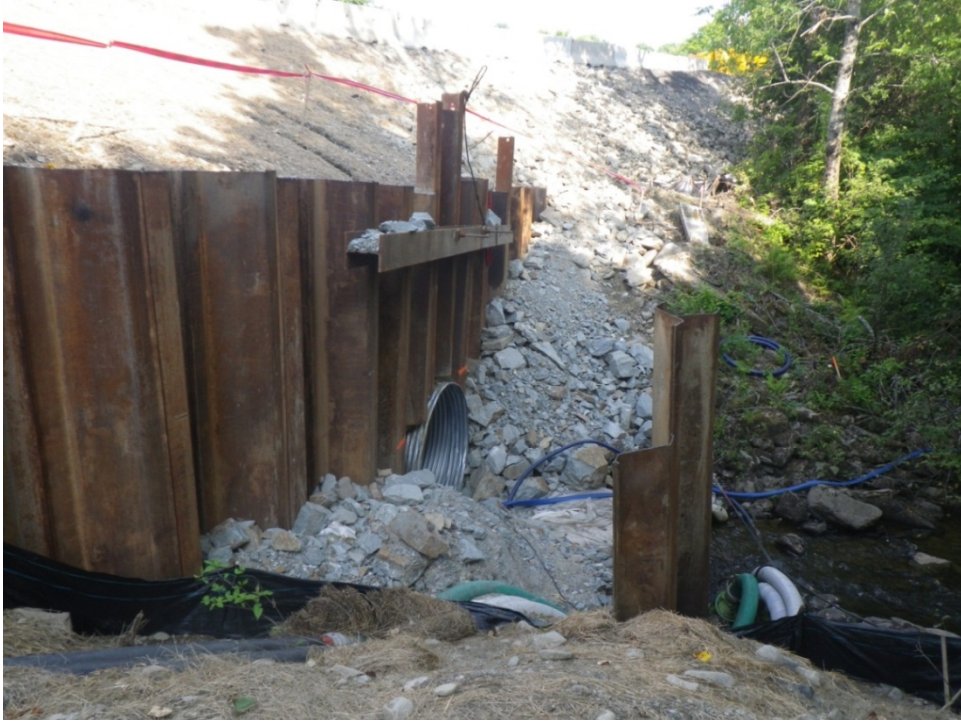
Sheet pile used as a cofferdam (upstream of work area).
