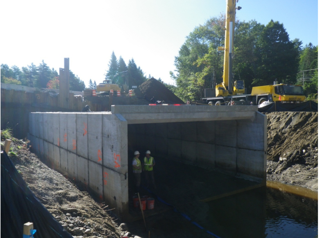
Concrete box culvert being set.
