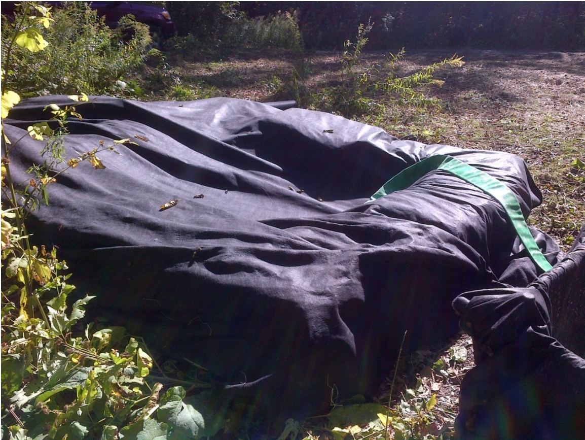
Hay bales and geotextile fabric used as part of a dirty water treatment system.
