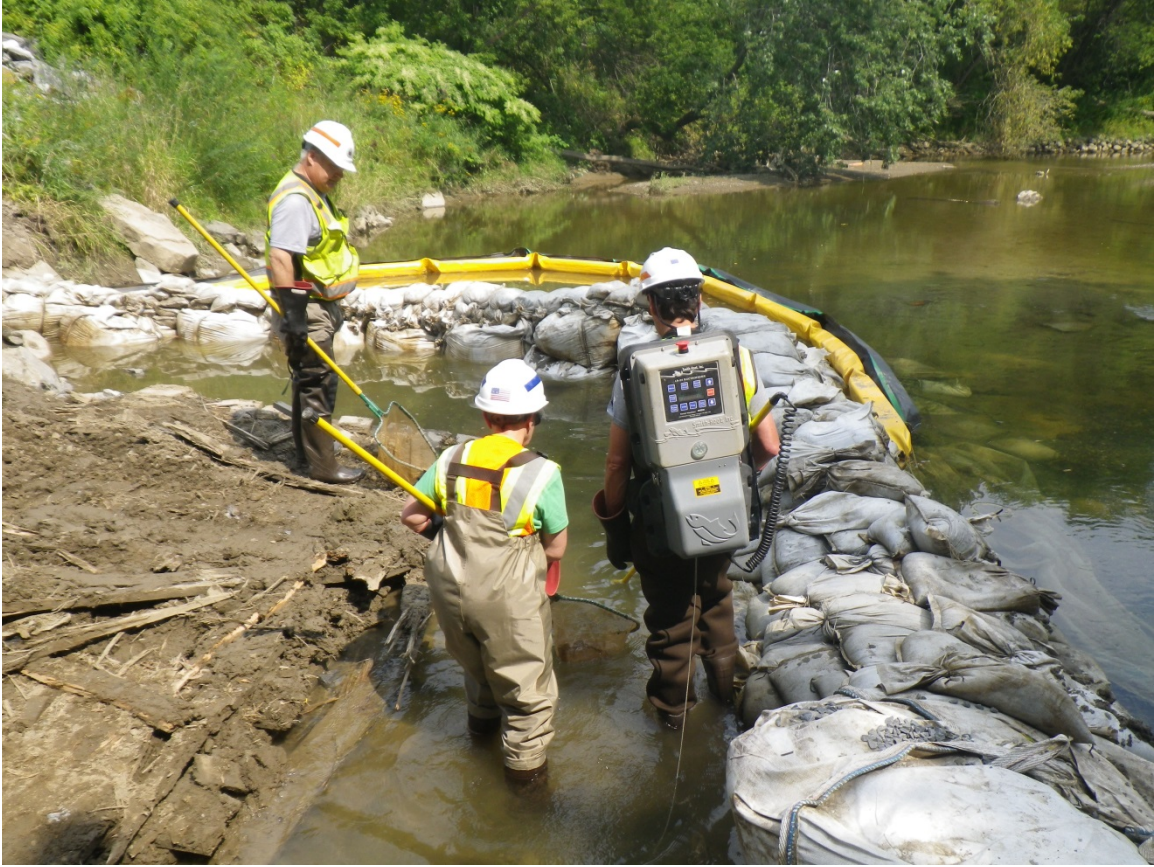
Example of a cofferdam constructed of small sandbags.
