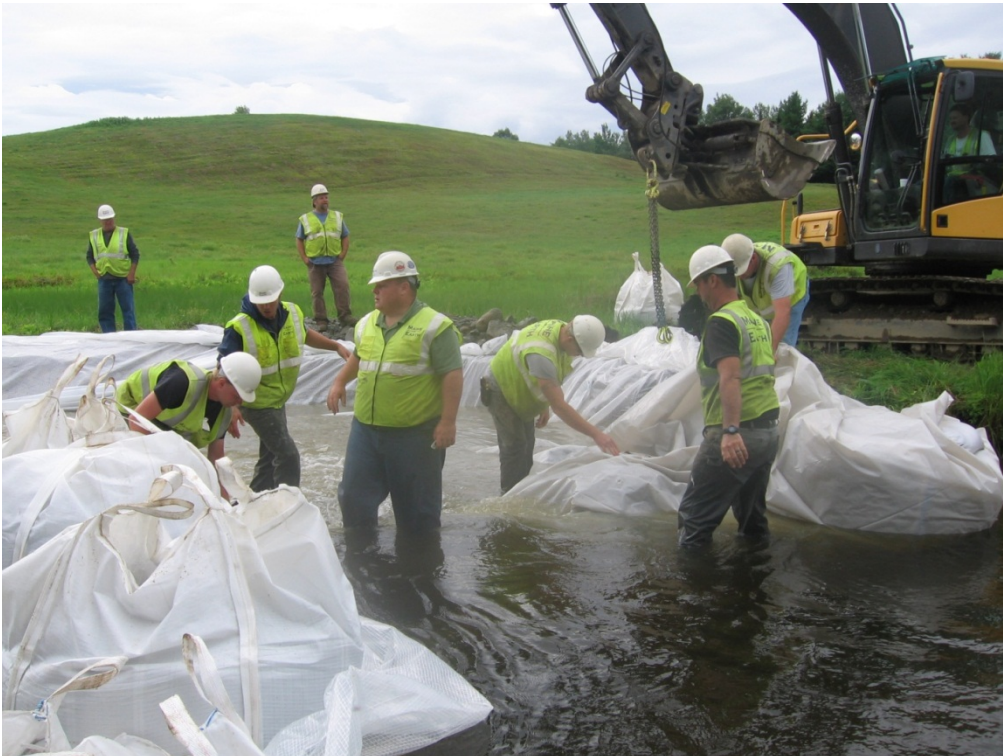
Placement of plastic sheeting under sandbag cofferdam.
