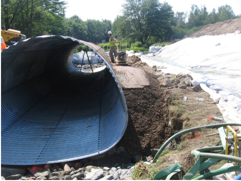
Crossing structure being 'bedded'.
