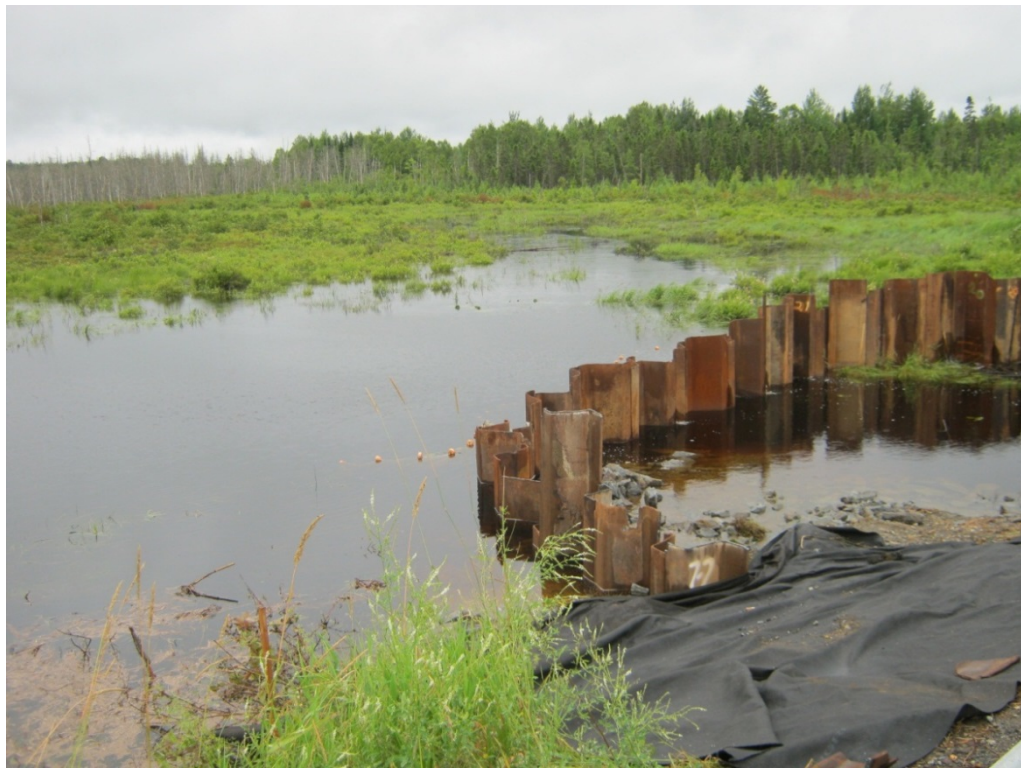
Sheet pile used as a cofferdam (upstream of work area).
