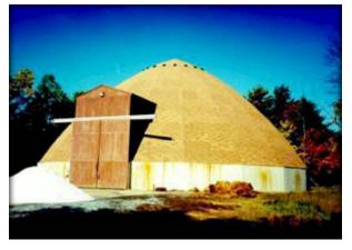
Dome, Concrete retaining wall, Wood Panels, Asphalt shingles
