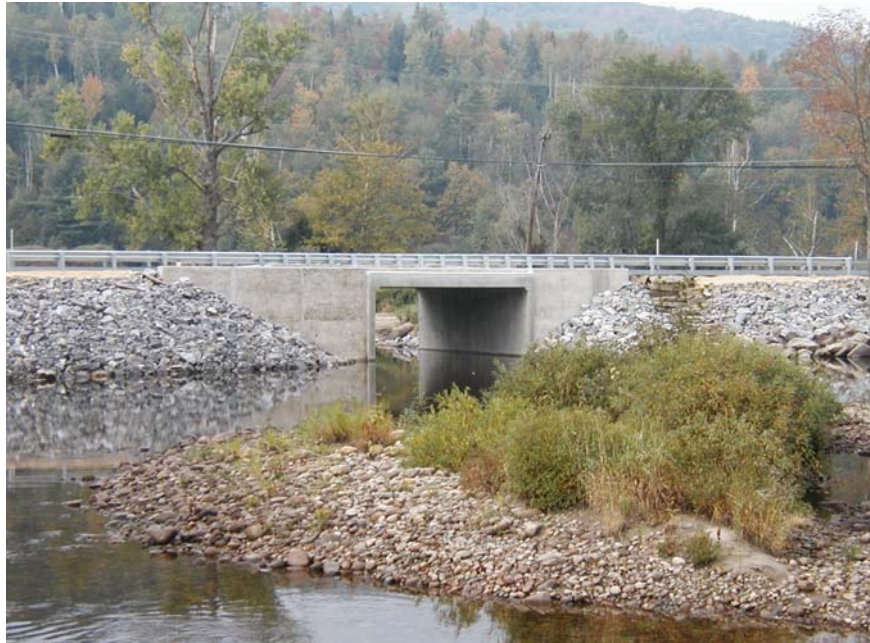
Scotty Richardson Bridge, Rumford
