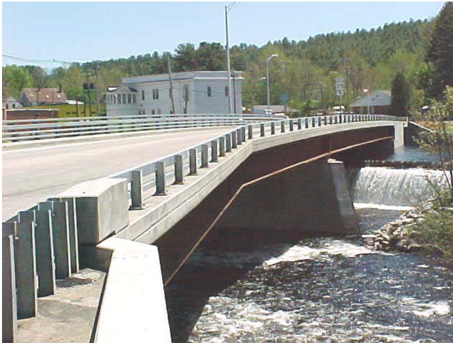
Kezar Falls Bridge, Parsonsfield-Porter
