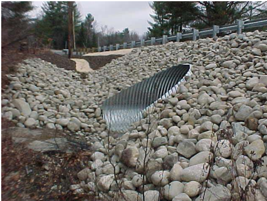
Twin # 2 Bridge, Farmington
