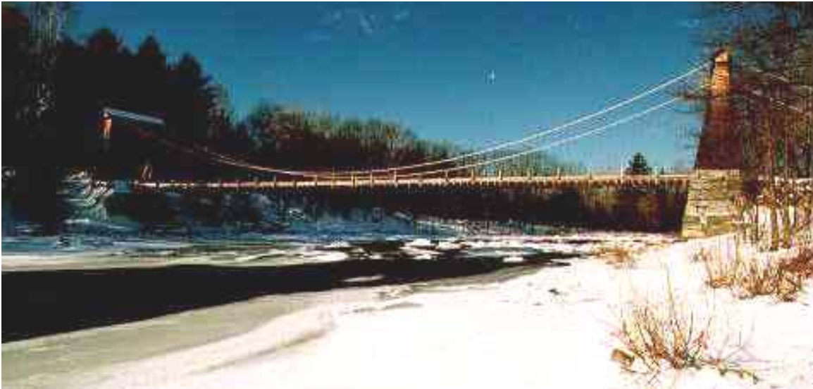
Wire Bridge, New Portland
