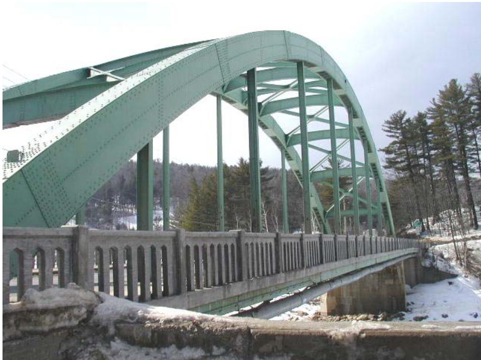
Morse Bridge, Rumford
