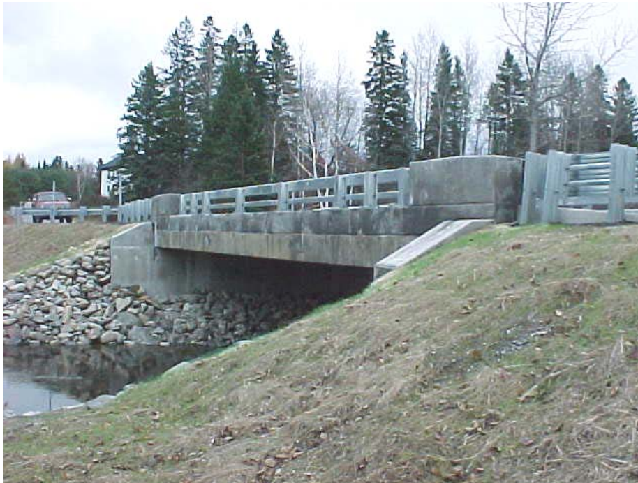
Sandy Stream Bridge, Moose River Plantation
