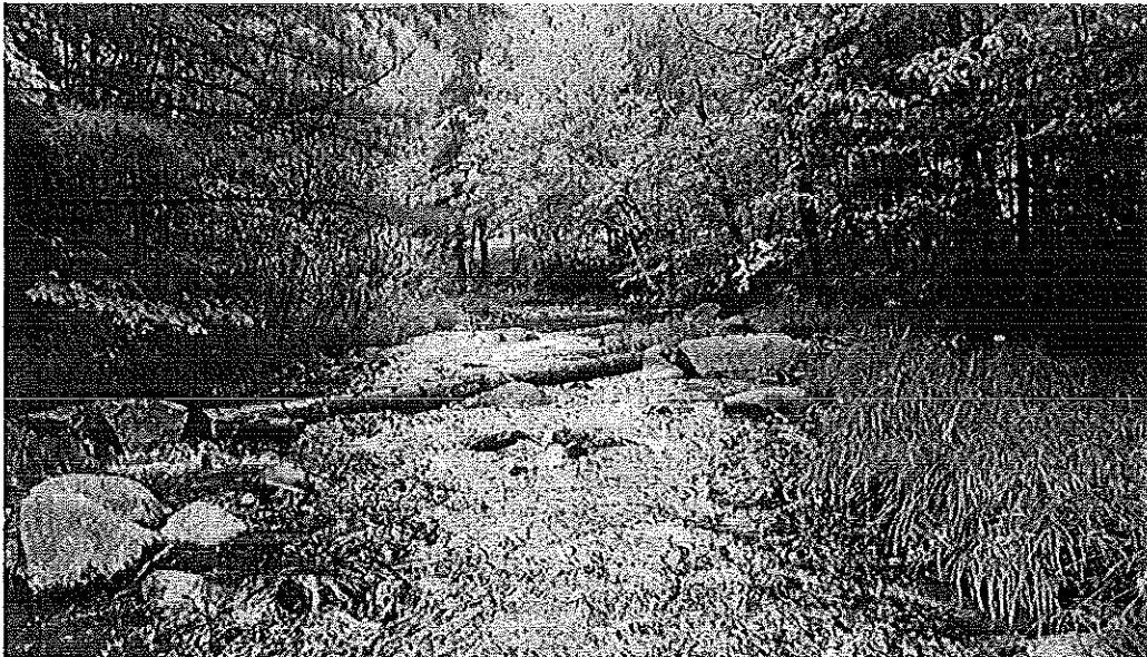
Transect 2 (Station 159, Project Area) looking upstream, September 2006, showing uppermost of 2 cabled logs placed diagonally to divert flow, thereby narrowing channel.
