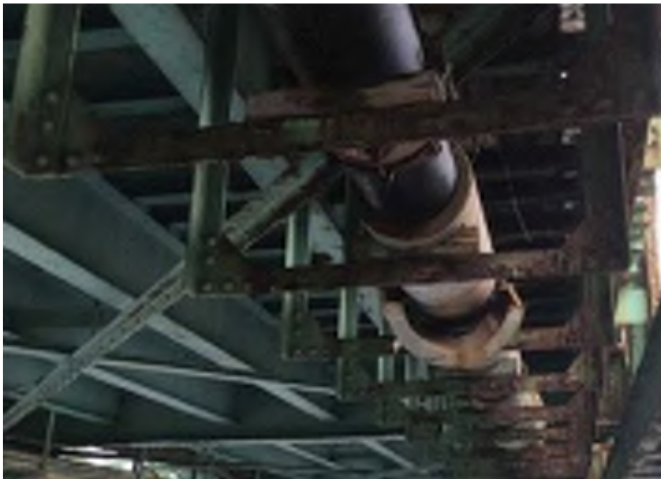
Figure 11: Bottom chord corrosion and debris
