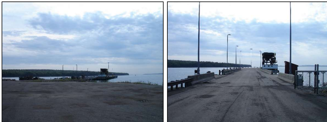
Figure 5: Mack Point Dry Cargo Pier 7
