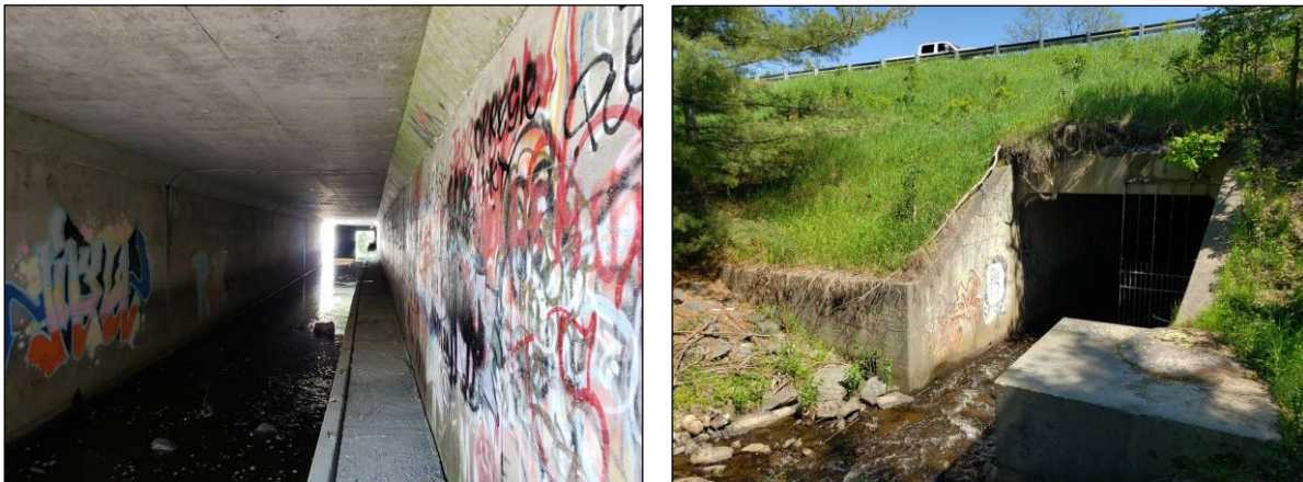
Figure 17, 18 The drainage culvert used by some to cross under I-95.
