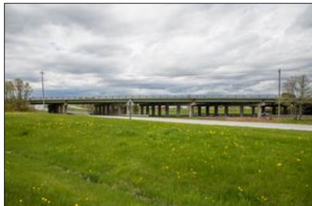
Figure 4 The Hogan Road Overpass.
