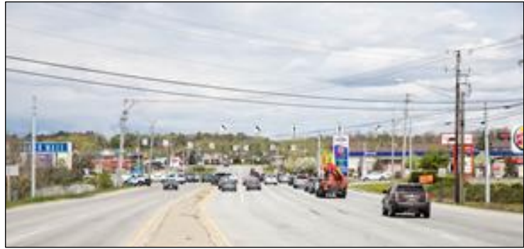
Figure 16 Hogan Road looking north just north of the overpass.
