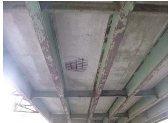
Approach Road Interchange Bridge – Over SB Lane
