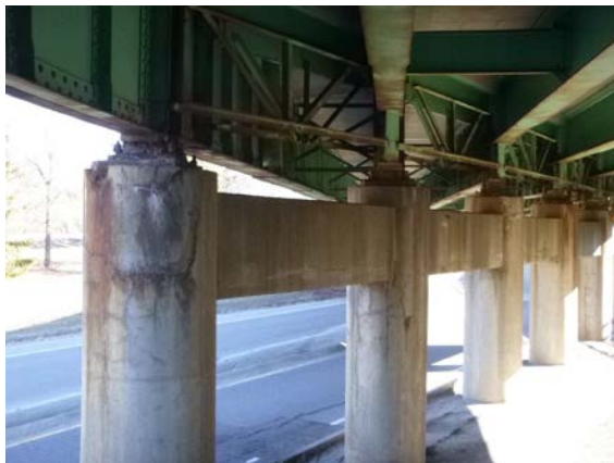
I-295 SB /Route 1 Bridge – South Pier
