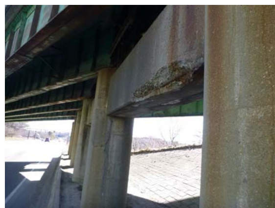
I-295 NB /Route 1 Bridge – South Pier
