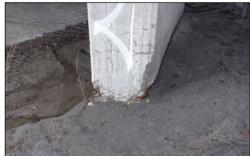
Above: Deterioration at center of east abutment. Below: Scaling at base of east pier, north end.
