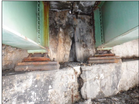
Above: Deterioration at center of east abutment. Below: Scaling at base of east pier, north end.
