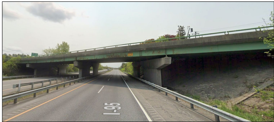
The Western Avenue Bridge in Augusta, Maine. Photo courtesy Google Maps.
