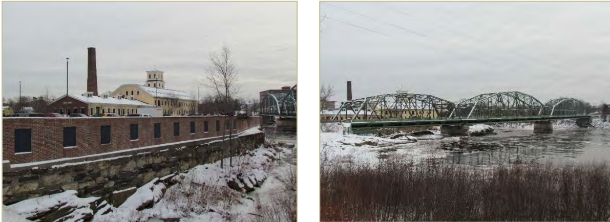
Figure 7. From Left to Right: Pejepscot Paper Company and Frank J. Wood Bridge
