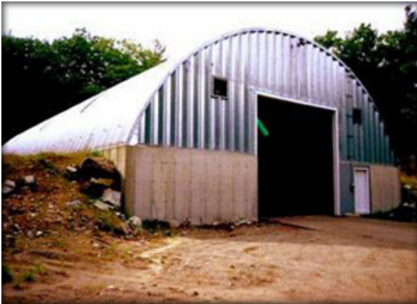
Metal arch, concrete foundation, bituminous paved floor
