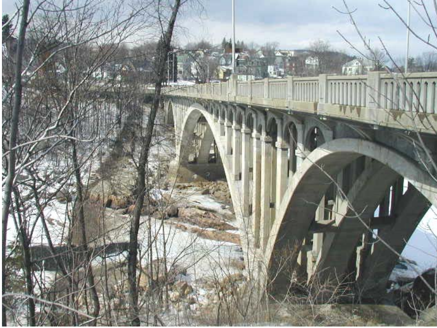
Chisholm Park Bridge, Rumford
