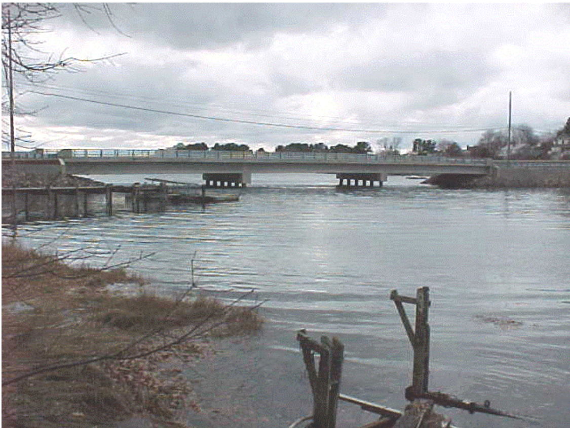
Kittery Point Bridge, Kittery
