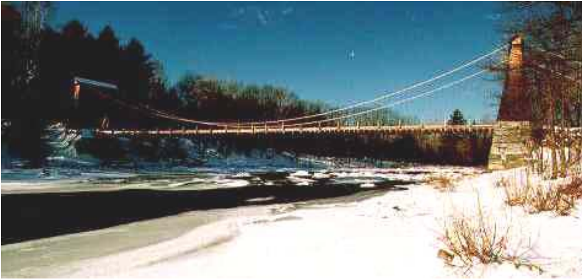
Wire Bridge, New Portland
