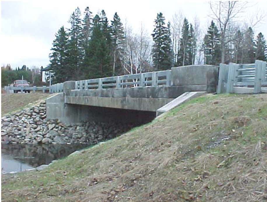
Sandy Stream Bridge, Moose River Plantation
