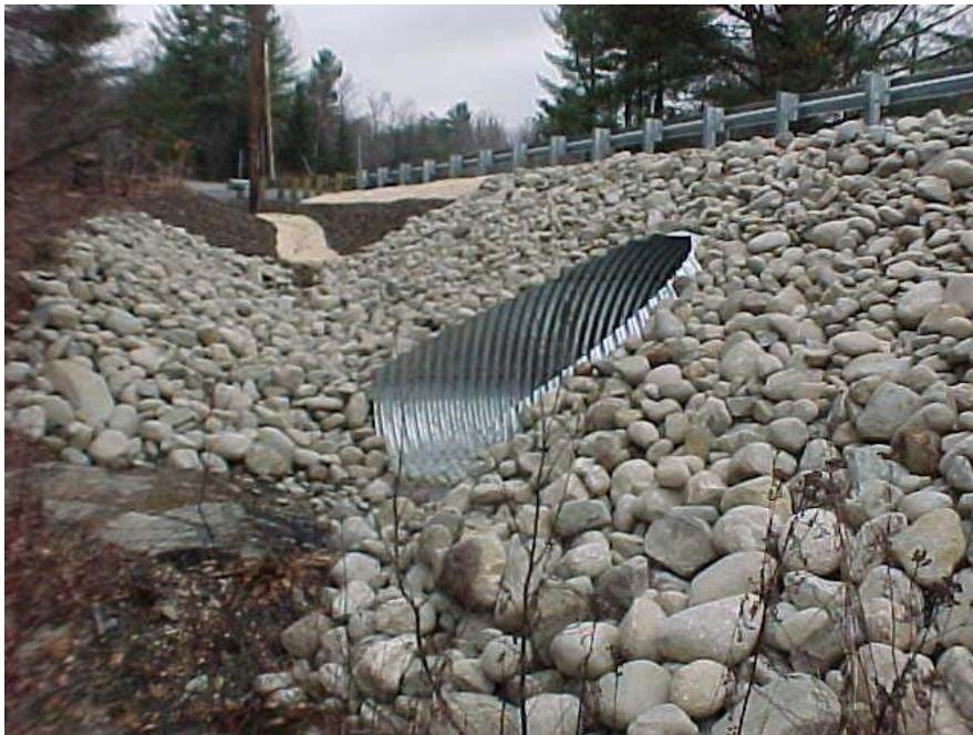
Twin # 2 Bridge, Farmington
