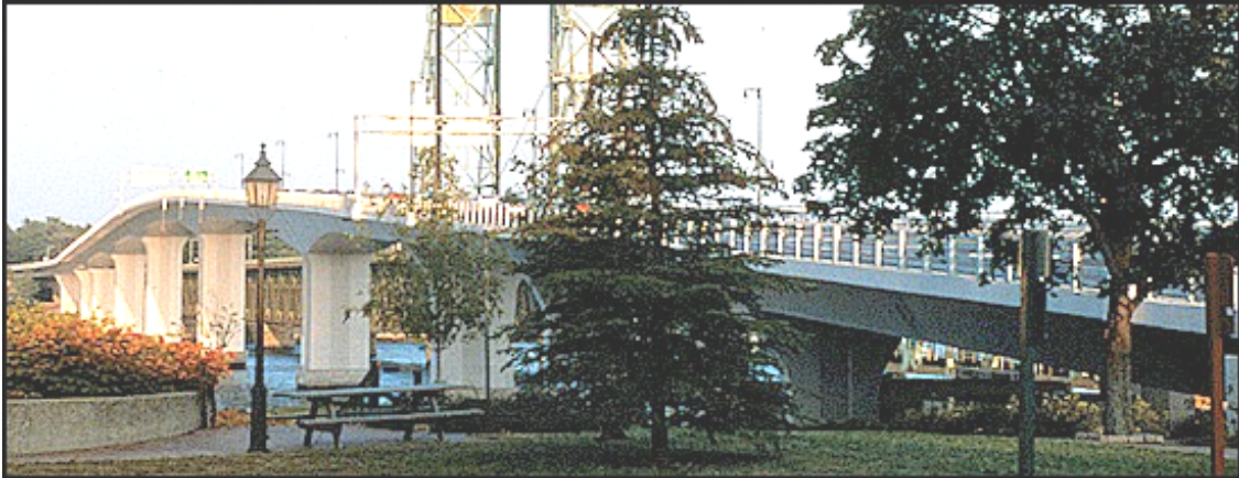
Sagadahoc Bridge, Bath-Woolwich
