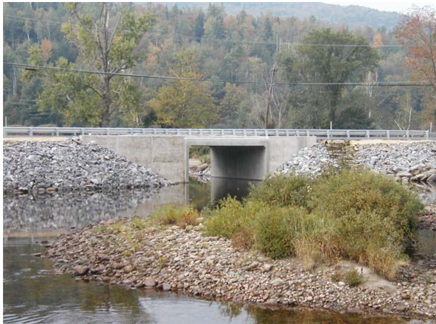
Scotty Richardson Bridge, Rumford
